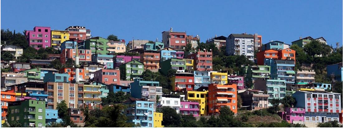
Figure 28. Facade painting work carried out in Samsun (URL 8).
