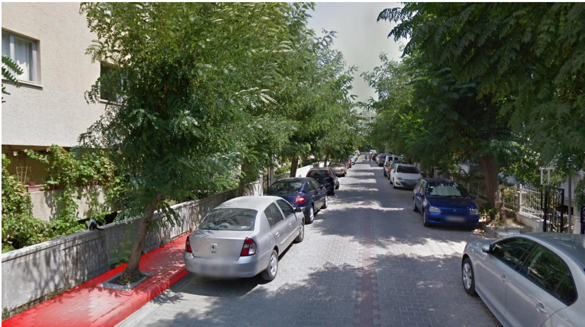
Figure 6.9. A sidewalk with insufficient width (50 centimeters) and obstructions in Bahçelievler Neighbourhood
