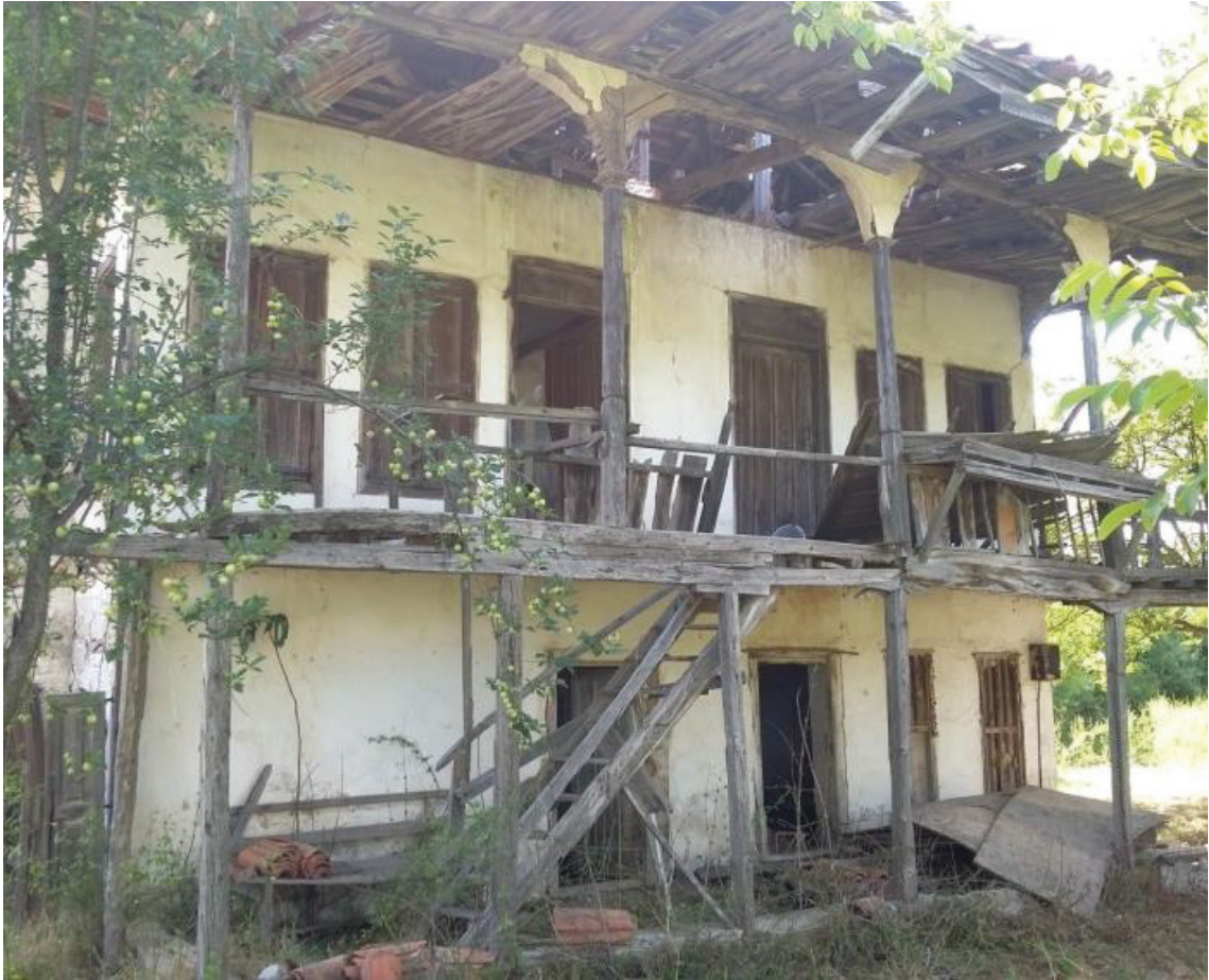
Figure 16. The building in Karabağlar, 208 block / lot 13 (front facade photograph)
