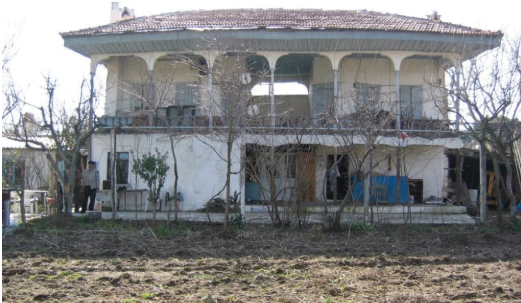
Figure 50. Sönmezer House north facade
