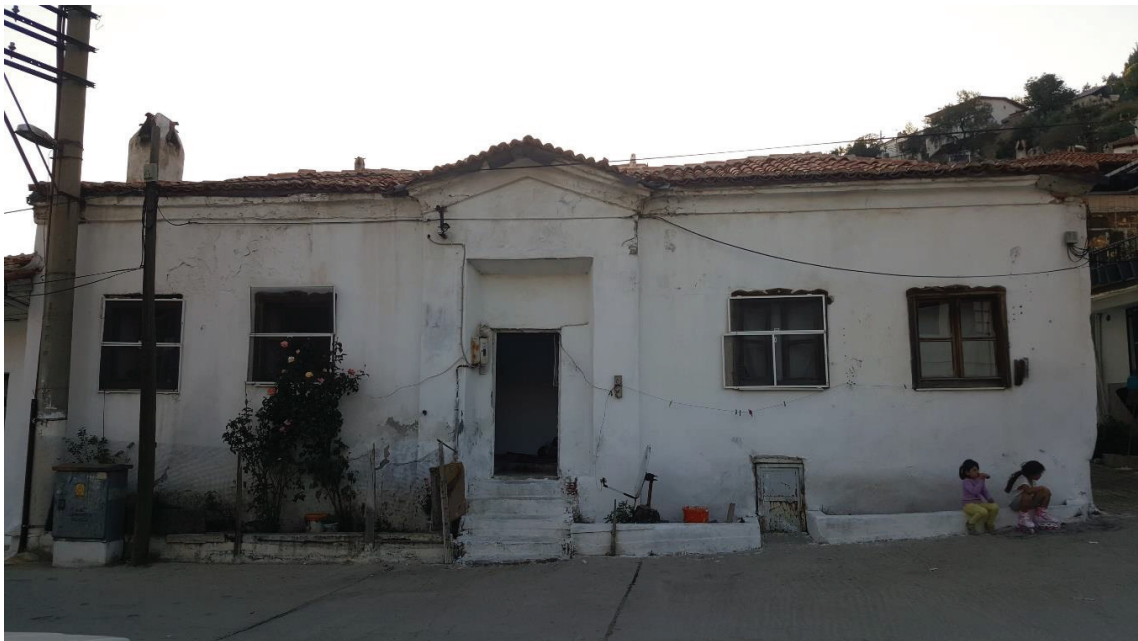
Photo 3.6. A registered building (a Greek architecture) in Saburhane (Source: Fulya Polat's archive 2019)
