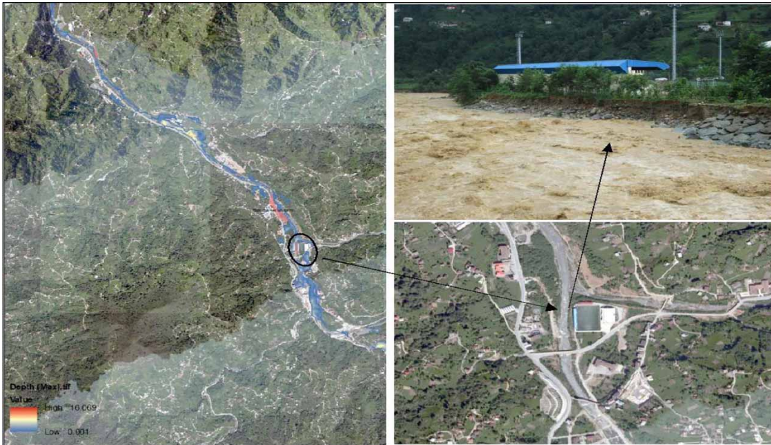
Figure 8 | Demolishing of the bank protection in the centre of the city.
