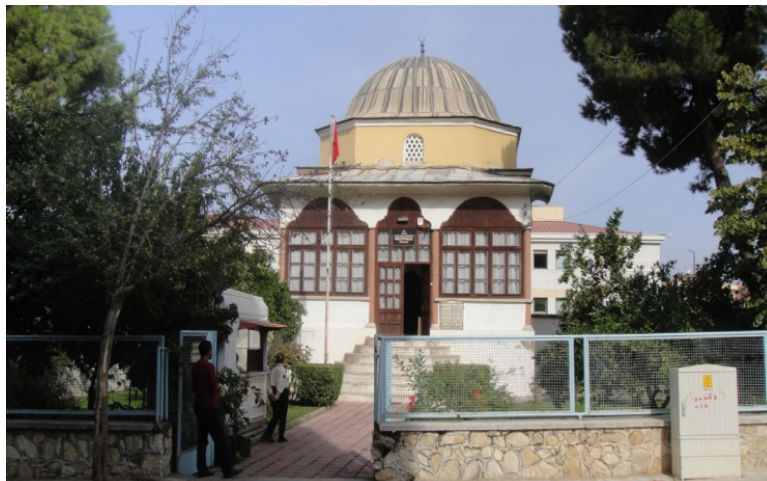
Figure 2 Entrance façade of the Necip Paşa Library (see online version for colours)
