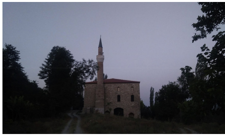
Fig. 4 Mosque mass, including its western entrance to a semi-open colonnaded space and its surrounding site.
