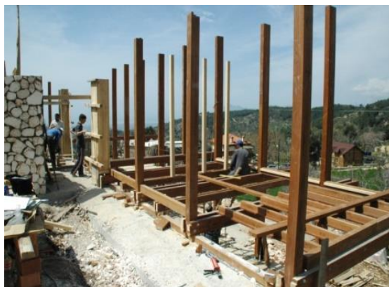
Figure 5.18. Column and Beam Laying
