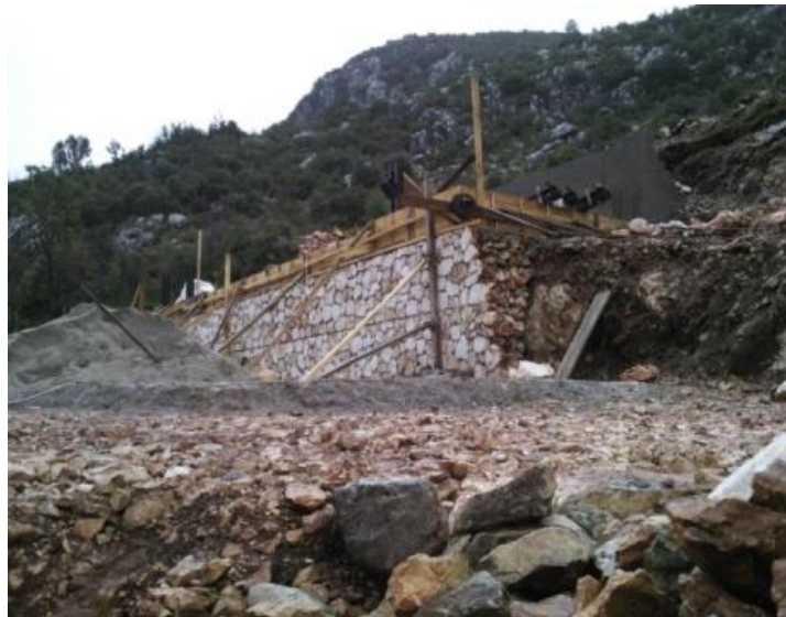
Figure 5.16. Retaining Wall Manufacturing
