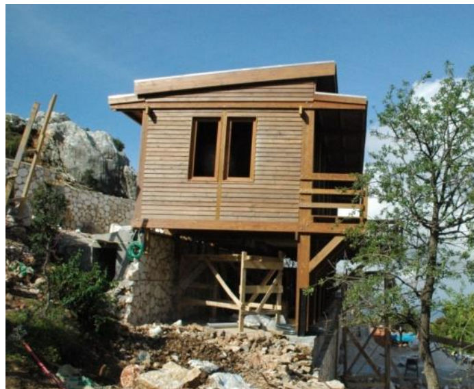
Figure 4. 18. JZ House Wall
