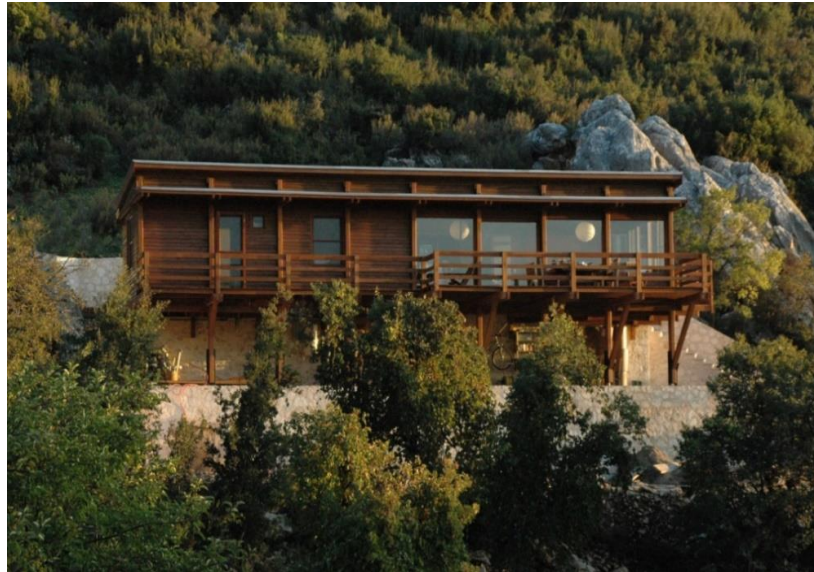
Figure 5.3. General View of JZ House
