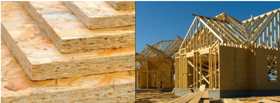
Figure 2.19. OSB Panel and Uses Example 23,24
