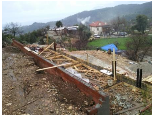
Figure 5.17. Preparation Stage for Foundation
