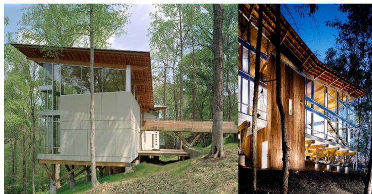
Figure 3. 1. Strickland-Ferris Residence, USA, 2008 31 .
