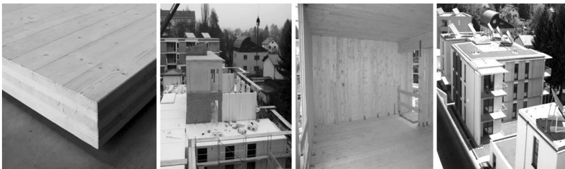
Figure 4. 8. (Left) Five-Layer CLT Element; (middle to right) Impressions From Project Wittenbauerstraße/Graz/Austria: Two Three-Storey Residential Buildings 44
