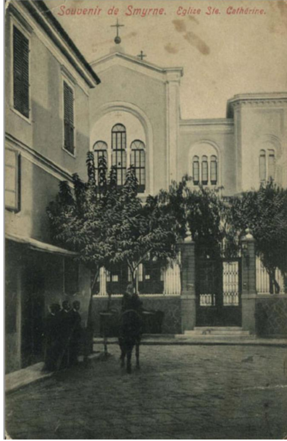
Figure 3.14. Agia Ekaterini quarter, south of Schoinadika (Pre-fire) ( Source: Levantine Heritage, 2019)
