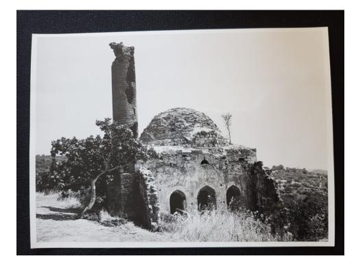
Figure 3.22. Mass collapse of minaret (dated on 1985) (Source: Ünal R. H personal archive)
