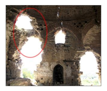
Figure 3.21. Mass collapse on the southeast part of the south wall of Harim
