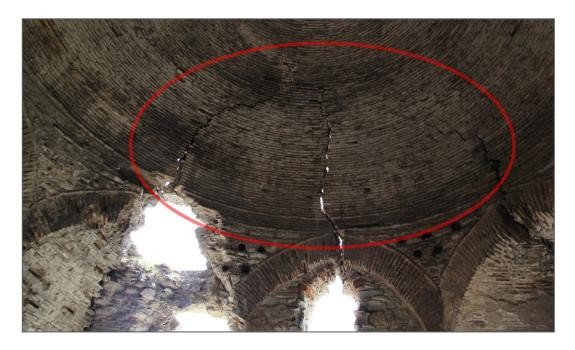
Figure 3.26. Crack on the south part of the dome
