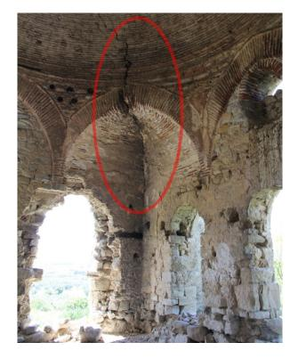
Figure 3.27. Cracks on the southwest corner of harim
