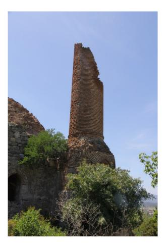
Figure 3.23. Mass collapse of minaret (dated on 2016)
