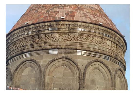
Figure 5.16. Steel tie bar application on the tomb of Çifte Minareli Madrasah in Erzurum
