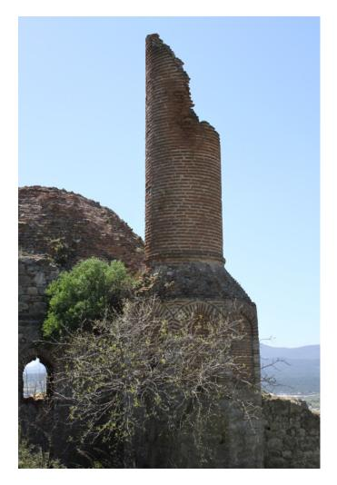
Figure 3.24. Mass collapse of minaret (dated on 2019)
