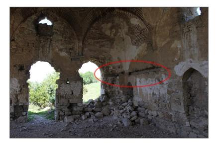
Figure 3.28. Loss of timber elements on north and west walls of harim
