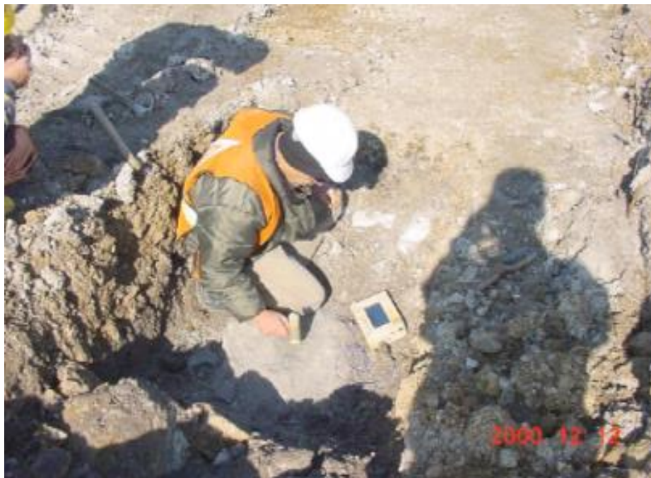
Figure 3.23. Sonic integrity test over the jet grout column (Gökalp and Düzceer 2000).
