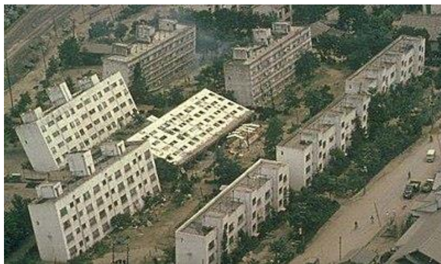
Figure 2.14. Loss of bearing capacity of buildings caused by liquefaction (Source: Niigata Nippo Newspaper, 1964).
