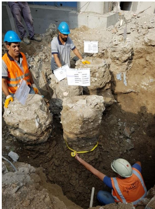
Figure 3.17. Discrete jetgrout columns.
