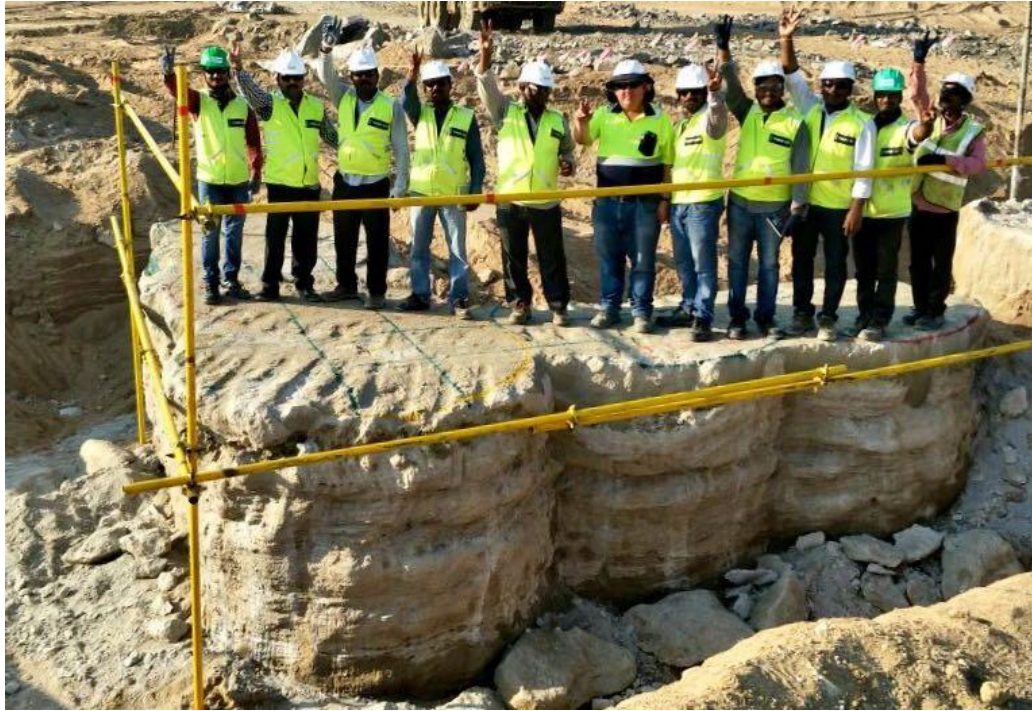
Figure 3.21. Test columns (Source: Kellerindia.)
