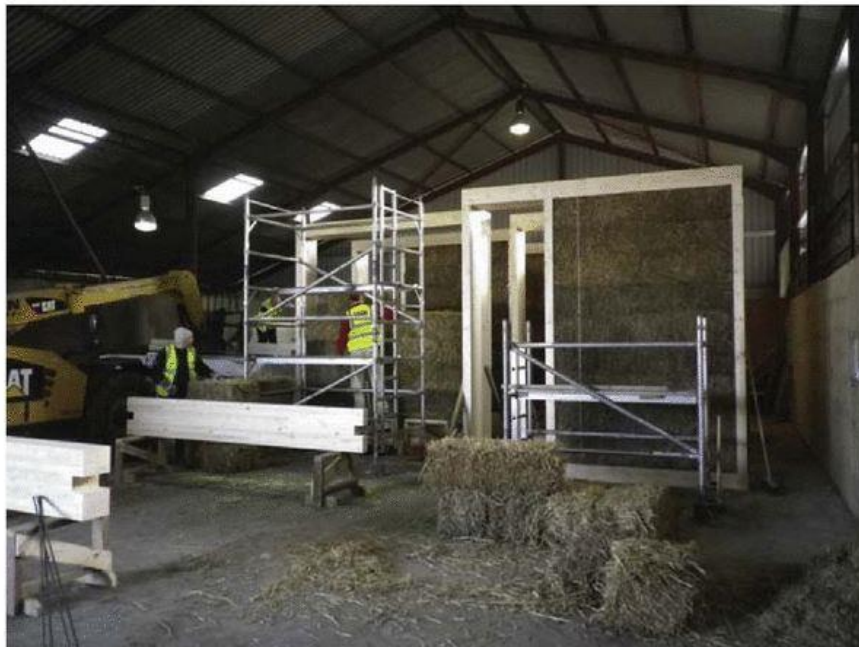
Figure 2.5. Fabrication of prefabricated straw bale panels (Source: Harries and Sharma, 2016)
