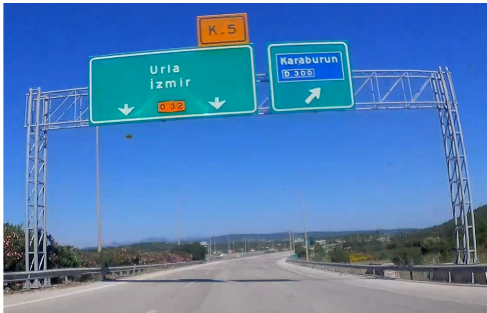
Figure 7. Motorway overhead directional information signs
