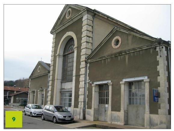
Figure 4. 24. Corner stones of Lyon Water Pump Station
