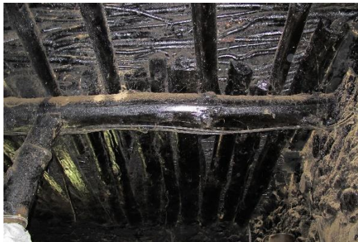
Figure 4.35. Ceiling of a house with tandır in Hişet village (June 23, 2017).
