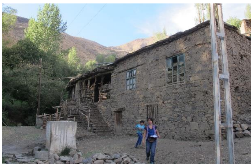
Figure 4.7. Abandoned dwelling unit of Faysal Bingöl (September 20, 2017).
