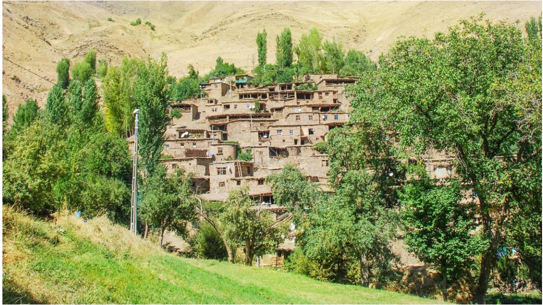
Figure 3.1. General view of Ahkis looking like one single integrated structure (Source: Nesiho Asiraki, 2011)
