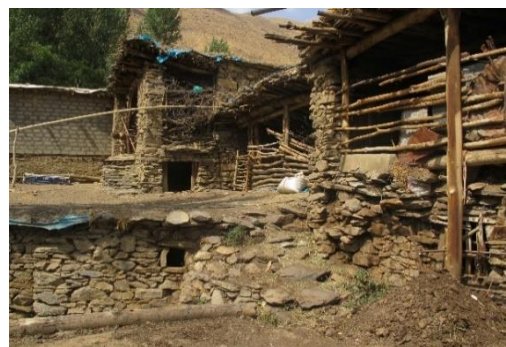
Figure 4.23. General view of Building group no. 3 (September, 2017).
