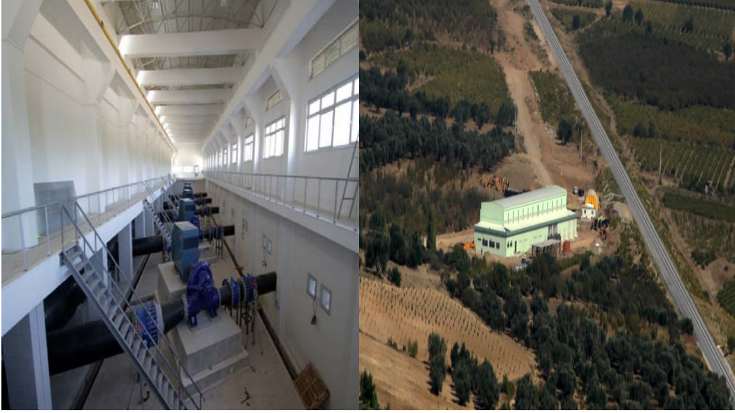
Figure 9.Çambel Pump Station
