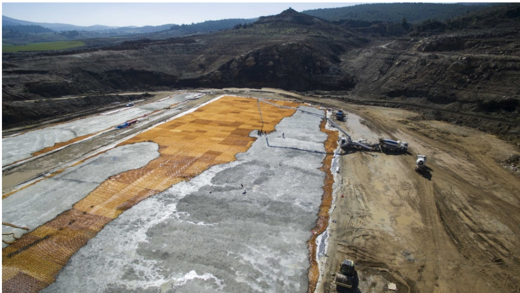
Figure 6. Gördes Ground Improvement
