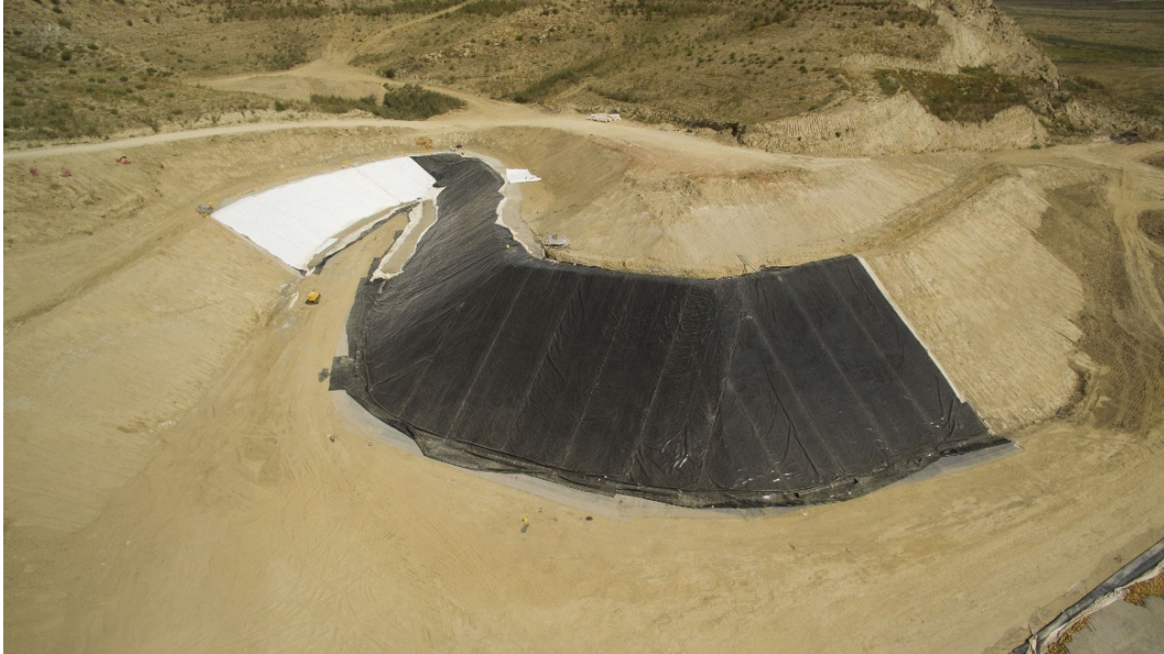
Figure 5. Gördes Ground Improvement
