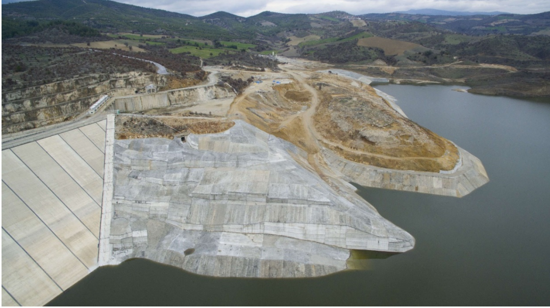
Figure 7. Gördes Ground Improvement
