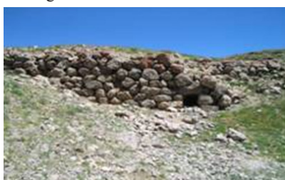
Figure 20 Ruins from Rusa Dam. 41
