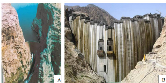
Figure 32 (A) Dez dam, height 203m, 54 years old in Khoozestan Province, (B) Karoon 4 dam, height 230m, 5 years old in Charmahal Bakhtiari Province.
