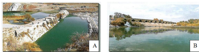
Figure 22 (A) Bahman weir dam. (B) Amir multi-purpose dam in Fars province.
