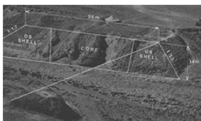
Figure 10 Sadd-Elkafara dam ruins and sketch for its cross-sectional dimensions. 25
