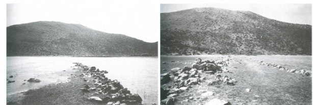
Figure 15 The Taka Dam as it can be seen today during winter and summer time. 35
