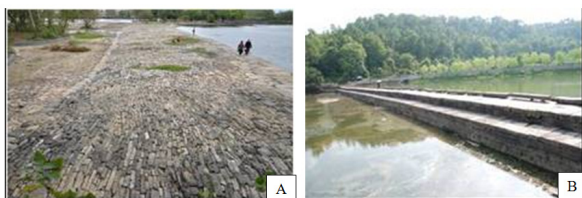
Figure 28 Ancient dams still in operation: (A) Part of the diversion dam in Lingqu canal, with part of the Xiang River left without water flow. By permission of A. N. Angelakis. (B) Tuo Shan Yan dam. 64
