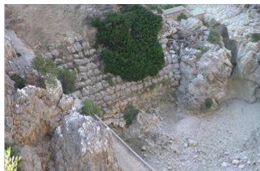
Figure 25 The dam of ancient Alyzia; general view and its spillway with its irregular shape formed by erosion through centuries (photo Angelakis AN).
