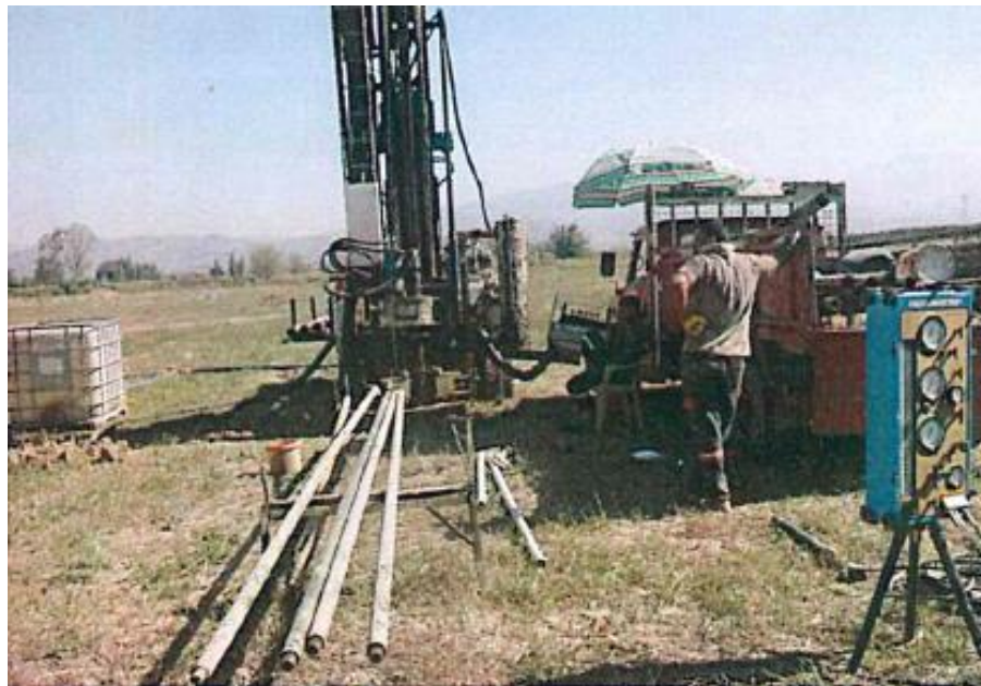
Figure 3.11. Application of PMT in The Geothermal Project
