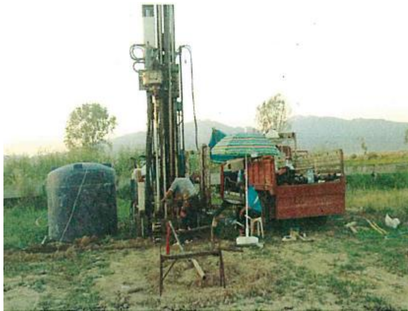
Figure 3.7. Standard Penetration Test in the Geothermal Project
