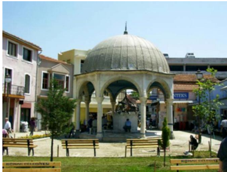
Figure 3.4: Ali Paşa Square after restoration studies (Source: İzmir Konak Municipality, 2005)
