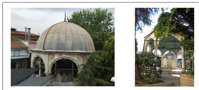
Figure 3.30: Fountain of Ali Paşa Square
