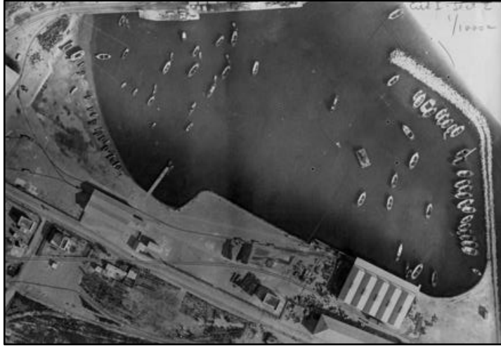
Figure 3.123. The aerial photos of the port area (Source: Kanbolat Archive)
