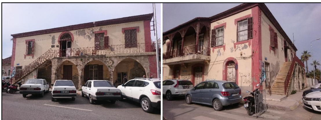
Figure 3.32. Syria Lebanon Bank (Date taken: 09.2018)
