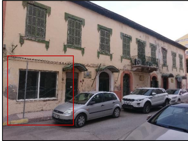
Figure 4.31. The British consulate building in today's İskenderun (Date taken: 09.2018)
