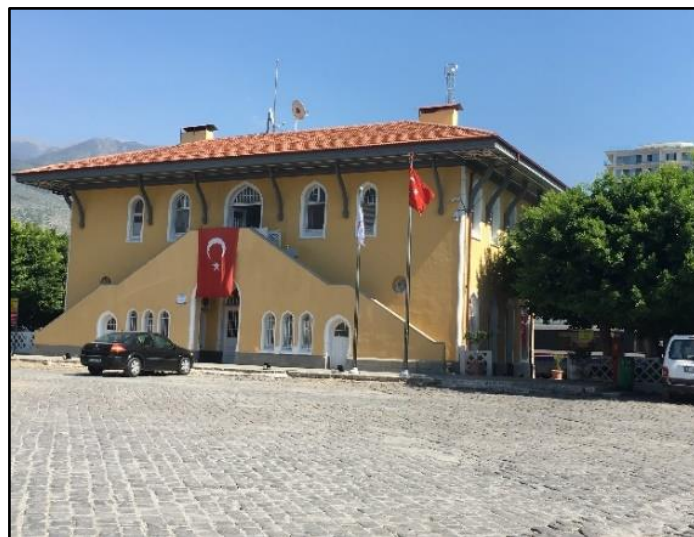
Figure 4.50. Station Building (Date taken: 09.2018)
