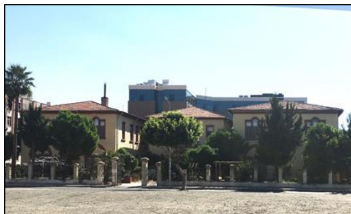
Figure 4.7. New Hospital in today's İskenderun (Date taken: 09.2018)
