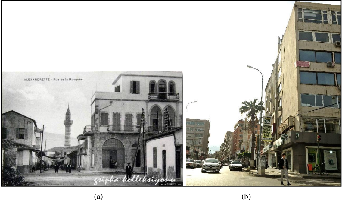
Figure 4. 14. (a) Sarraf Hotel in Mandate period (Source: wowturkey, “İskenderun.”) (b) Environment of Sarraf Otel in today’s İskenderun (Date taken: 09.2018)
