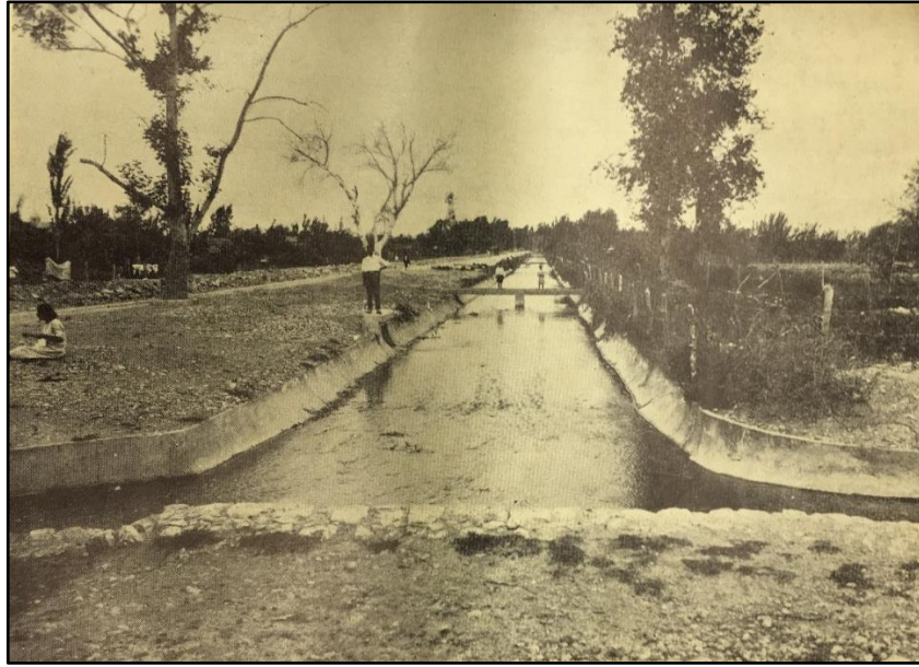
Figure 3.80. Reinforced concrete channels
