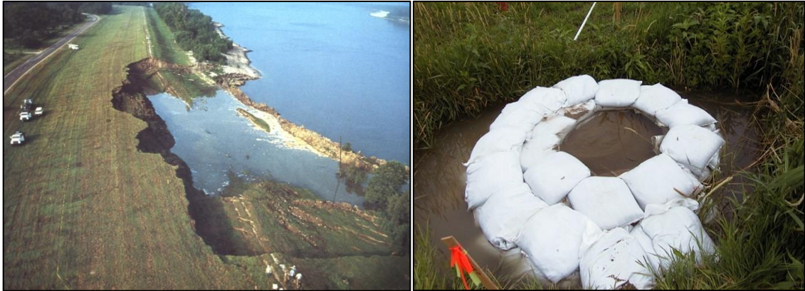
Figure 2.3 Erosion and Sand Boil formations Mississippi and Louisiana river levee (Source: Sherman 2008)
