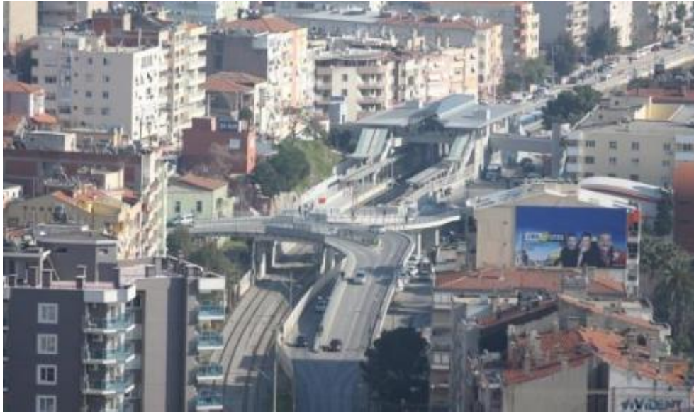
Figure 49. Bayraklı İZBAN Station (Railway) (Source: www.bayrakli.bel.tr , 2017)
