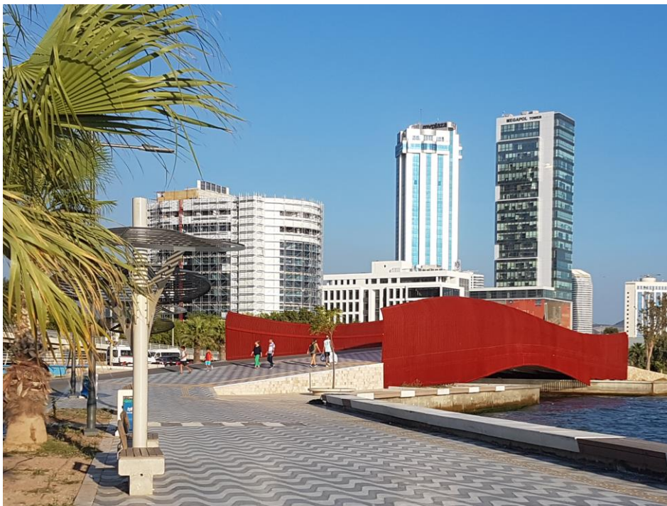
Figure 54. Footbridge on Bayraklı Seashore (Source: Photo taken by Author, 2018)
