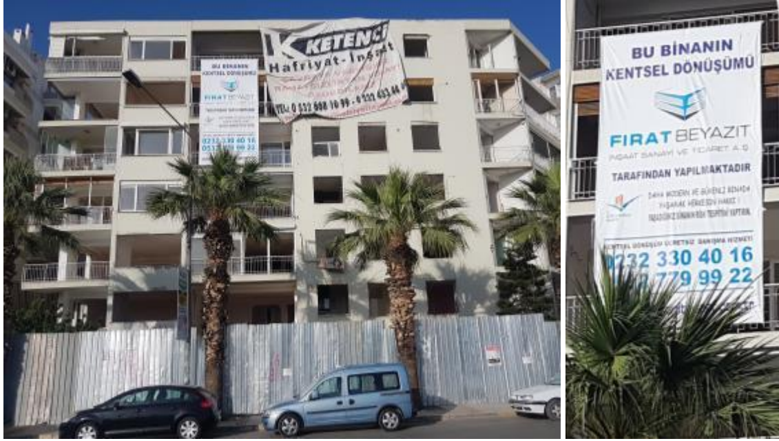
Figure 1. Rebuilding in Bostanlı, İzmir. (Source: Photo taken by the author, 2018)
