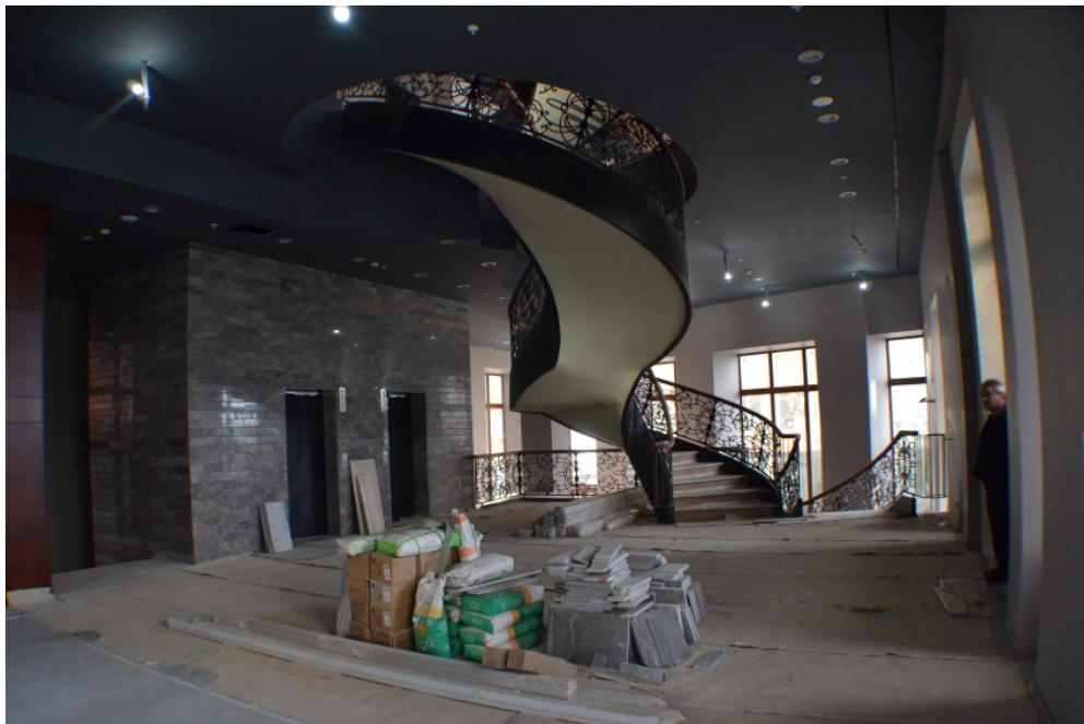
Figure 3.20. The interior of Frej Apartment Building in restoration, 2016.
