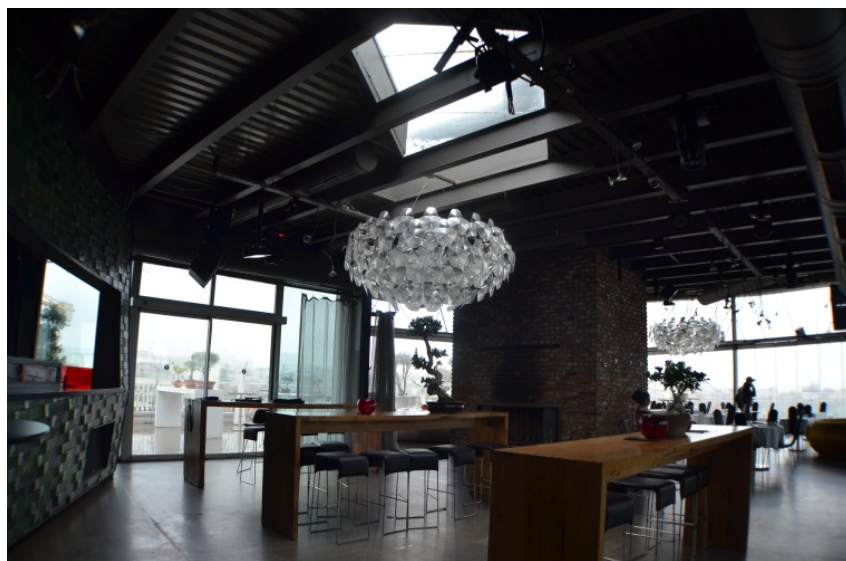
Figure 3.34. Steel structure of the roof restaurant called 360, 2016.
