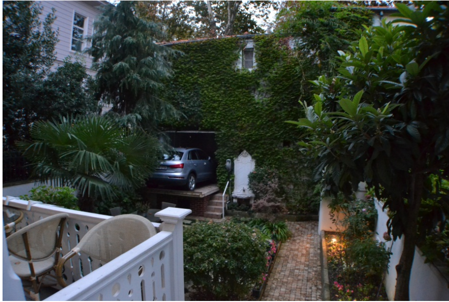
Figure 3.12. The courtyard of Faik Bey Yalı and block 316, lot 4 at the left, 2016.
