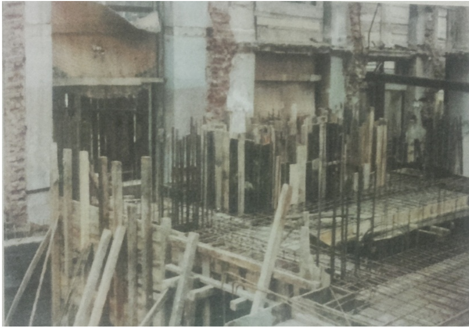
Figure 3.19. Frej Apartment in 1987-88 during the renewal work, interior structure completely changed and only façade was conserved as a shell (Source: Onat, 1989, cited in Tanyeli, 2012).
