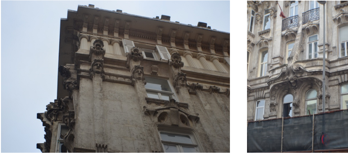
Figure 3.28. Detail photos of the facade of Gümüşsu Palas, 2016.
