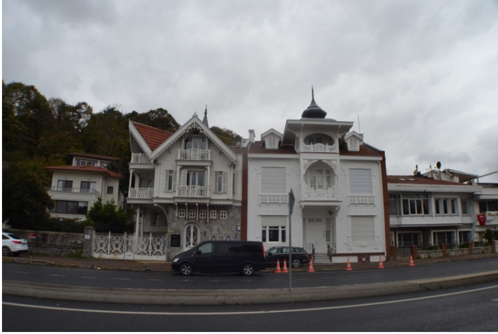
Figure 3.2. Dikranyan Yalı and adjoining buildings as viewed from the seaside, 2016.
