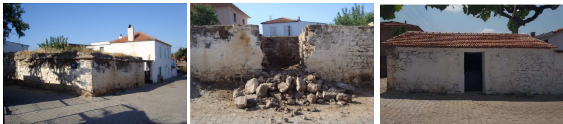
Figure 80. Alteration of earthen flat roof into gable one. 2017.
