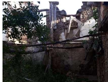
View from ground level.
