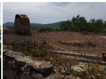
Earth roof, April 30, 2017
