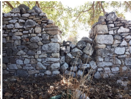
Door opening. September 23, 2017.
