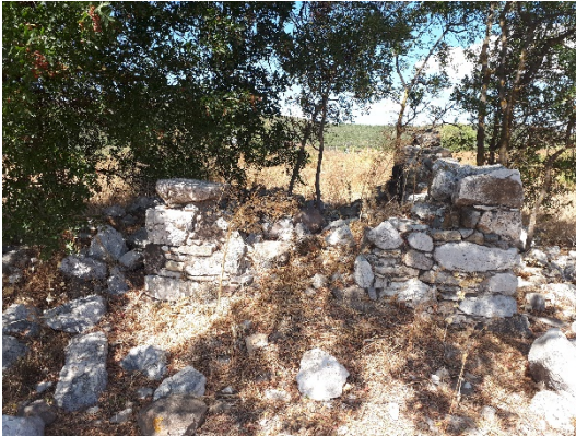
Ruined house. September 23, 2017.
