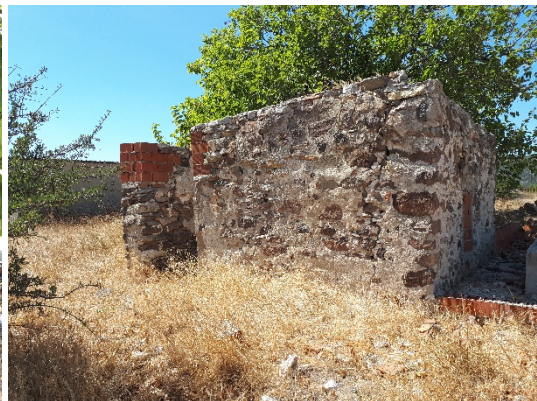
Door opening. September 23, 2017.
