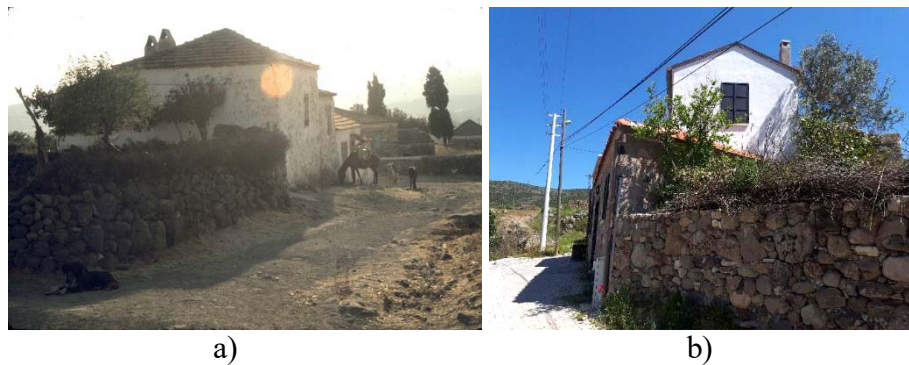
Figure 102. a) Brushes on top stonewall. (Source: Erzen, J. n.d.) b) Brushes on top stonewall. (April 26, 2017)
