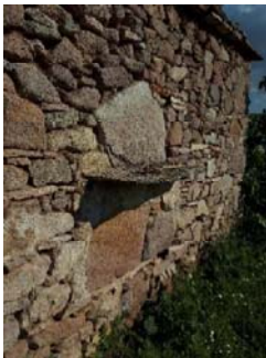
Exterior of the niche, slate stone shelf
