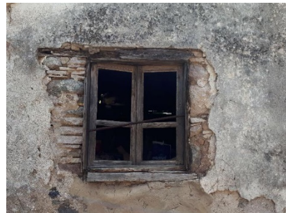
Wooden window frame
