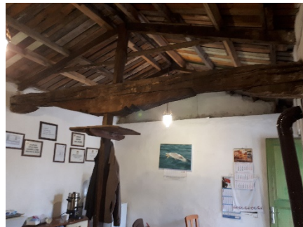
Wooden column, beam, transition elements, direkbaşı .
