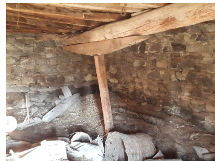
Wooden column, beams, transition elements
