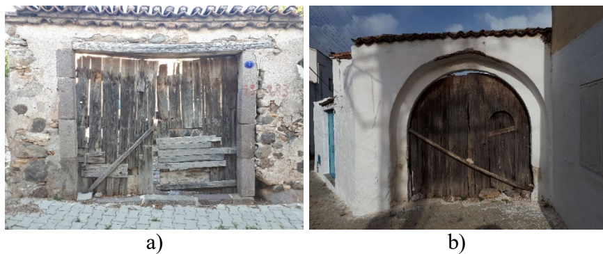
Figure 56. a) Rectangular courtyard door. April 26, 2017. b) Arched top courtyard door having sash in a sash. May 9, 2017.
