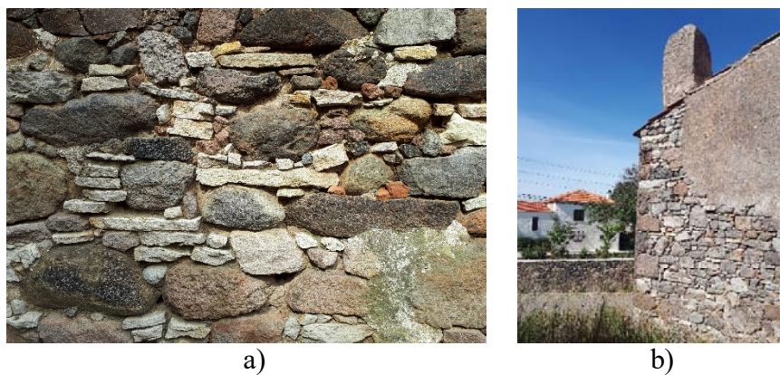
Figure 60. Wall bondings. a) March 13, 2017. b) April 25, 2017.
