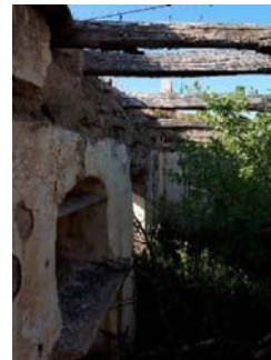
Wooden roof beams
