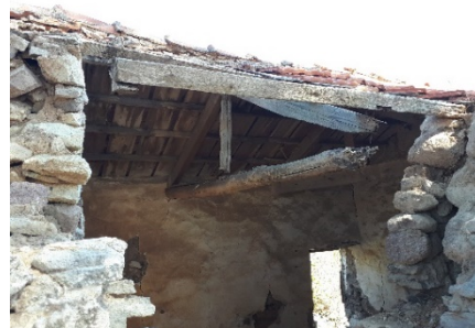
Roof structure. September 23, 2017.
