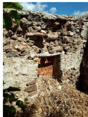
Window opening. September 23, 2017.
