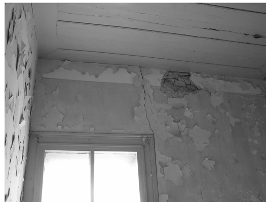
c and d) Deteriorated wall section at the north-east corner due to the crack that permits moisture to penetrate
