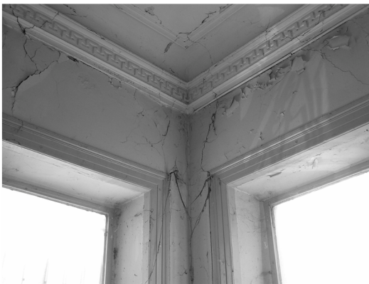
e and f) Typical cracks at the top of the windows
