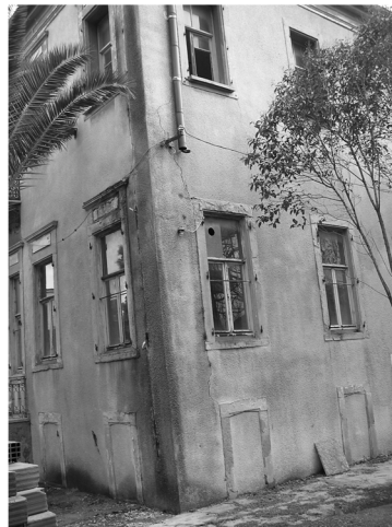
c and d) Deteriorated wall section at the north-east corner due to the crack that permits moisture to penetrate
