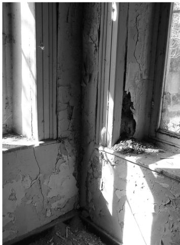
c and d) Deteriorated wall section at the north-east corner due to the crack that permits moisture to penetrate
