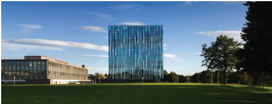
Figure 2.9. Exterior view of the University of Aberdeen New Library. (Source: http://www.archdaily.com/276161/university-of-aberdeen-new-library-schmidt-hammer-lassen-architects )
