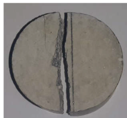
(b) Crack profile
