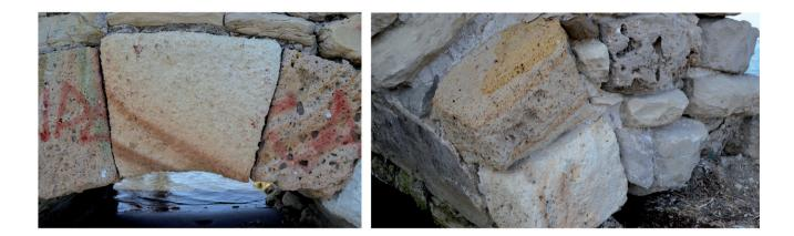
Figure 9. Lime mortar connecting voissours with each other and spanderal wall
