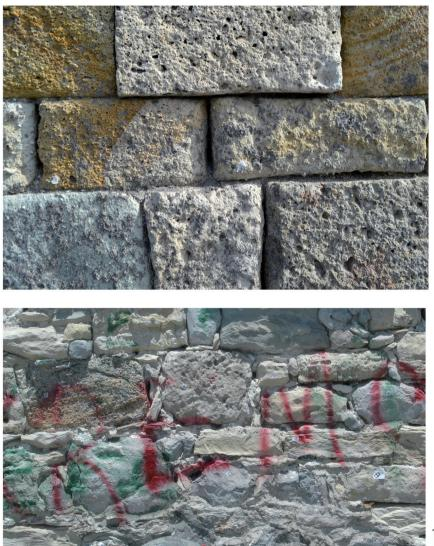
Figure 8. Differences between the outer shells a) Outer shell on the coastside: Rough cut limestone with broad joints, b) Outer shell on the seaside: Cut sandstone blocks with close joints a
