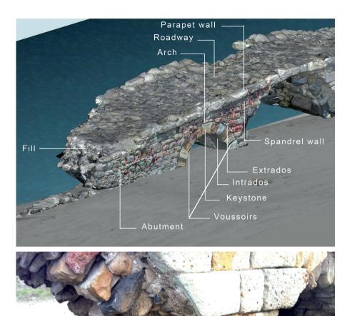
Figure 5. Elements of the Hypokremnos Bridge, axonometric view from the 3D survey model
