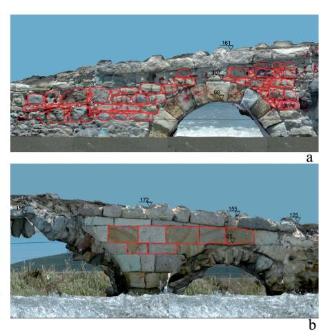
Figure 7. a) Upstream (Southwestern) Façade, b) Downstream (Northeastern) Spandrel walls, orthogonal views from the 3D survey model
