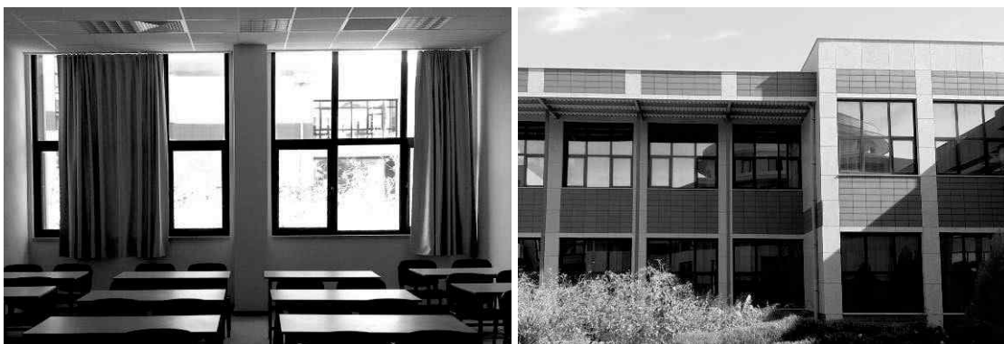
Fig. 1. Interior and exterior views of windows in Room B
