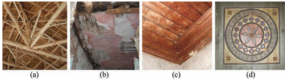
FIG. 24. (a) Roof truss with hanging post (Tire-Kızılcahavlı) and ceilings with: (b) reed matting with plaster (Bergama-Sarıcalar), (c) planks (Çeşme-Ildırı), and (d) ornaments (Bergama-Sarıcalar).
