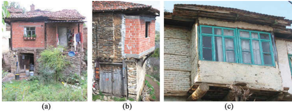
FIG. 26. Spatial changes with: (a–b) RC slab and hollow bricks walls (Beydağ-Alakeçili), and (c) window enlargement of a bay window in humiş frame with brick infill (Kiraz-Karaburç).
