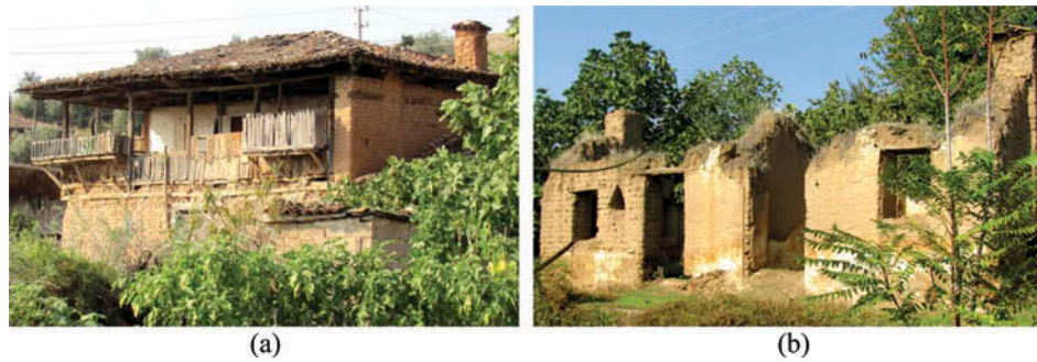
FIG. 10. (a) A double-story adobe brick masonry house; (b) remains of an adobe brick masonry house (Ödemiş-Alaşarlı).
