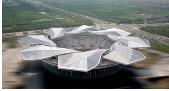
Figure 2.24. Qizhon's Retractable Roof (Source: www.isaarchitecture.com )
