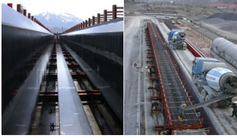
Figures 3, 4: Precast beam production.
