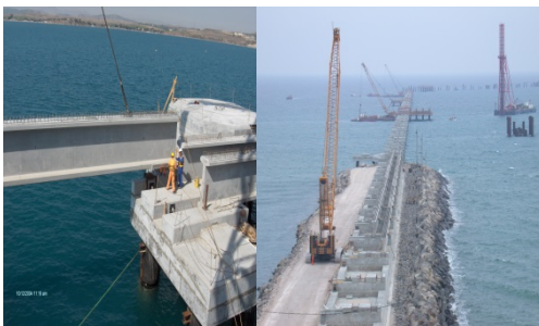
Figures 9, 10: Precast beam installation.
