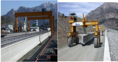
Figures 5, 6: Precast beam delivery.
