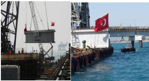
Figures 7, 8: Precast beam installation.
