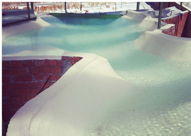
Fig. 2. View of the dam reservoir
