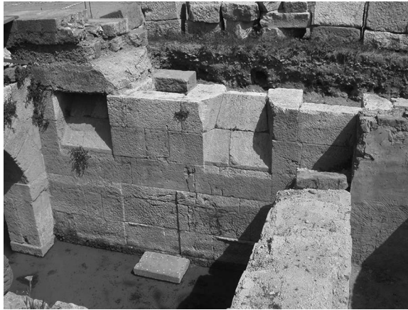
Figure 10. Photograph of the east wall after removal of the 1930s reconstruction.
