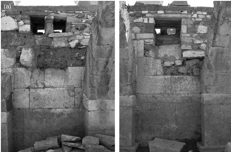
Figure 9. Photograph of the 1930s reconstruction of the slit window and the crepidoma: a) The reconstruction between the tenth and eleventh abutments; b) The reconstruction between the fifteenth and sixteenth abutments.
