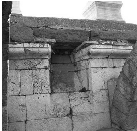
Figure 5. Photograph of slit window and stringcourse on the east wall (seventh and eighth abutments).
