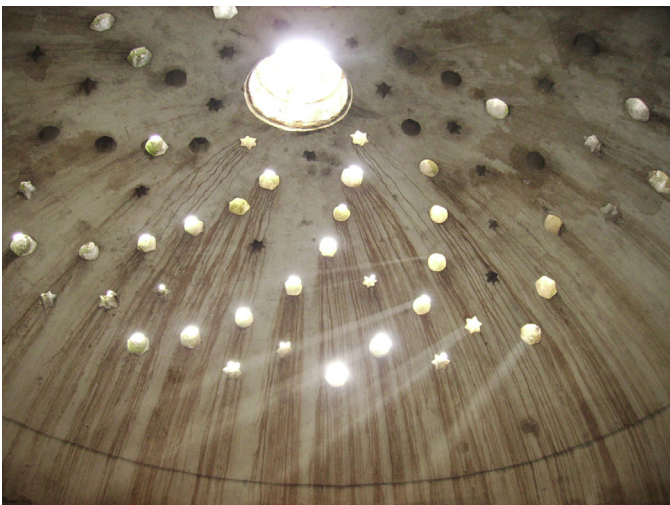
Fig. 2. The interior view of Yalınayak Bath hot main space dome, hexagonal oculi in spiral geometrical order with star shaped in between randomly.
