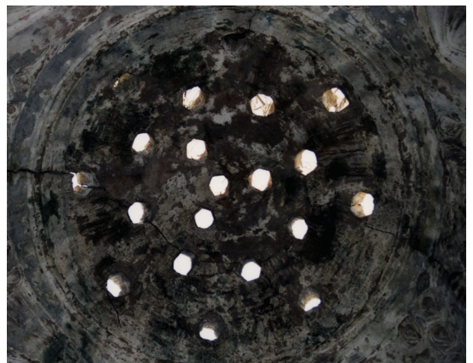
Fig. 10. The east hot room dome of Urla Kamanlı Bath, use of hexagonal shaped oculi formed by brick bond in circular three rows.
