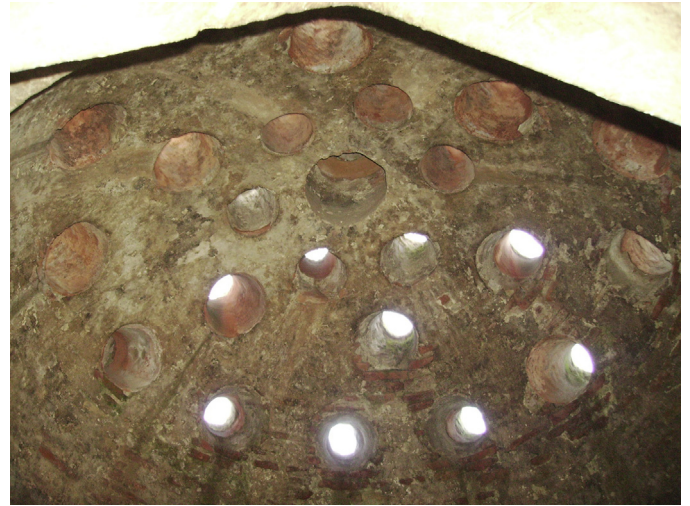
Fig. 9. Tire Hekim Bath men's section southeast hot room dome, use of terracotta pipes in the brick bond.
