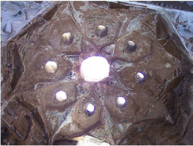
Fig. 1. The interior view of Tahtakale Bath iwan dome, hexagonal oculi in overlapping geometric pattern.
