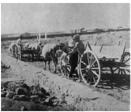
Figure 1. The villagers working at a school construction (Köy Okulu Binası, 1937). Close examination of the photo reveals that women also worked at constructions. Right in front of the building, a woman is mixing mortar with a shovel, and other women are carrying construction materials to the building and other places as needed.
