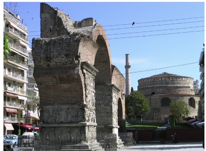
Fig. 2. Galerius Palace complex: The “Rotunda” and the “Kamara”.
