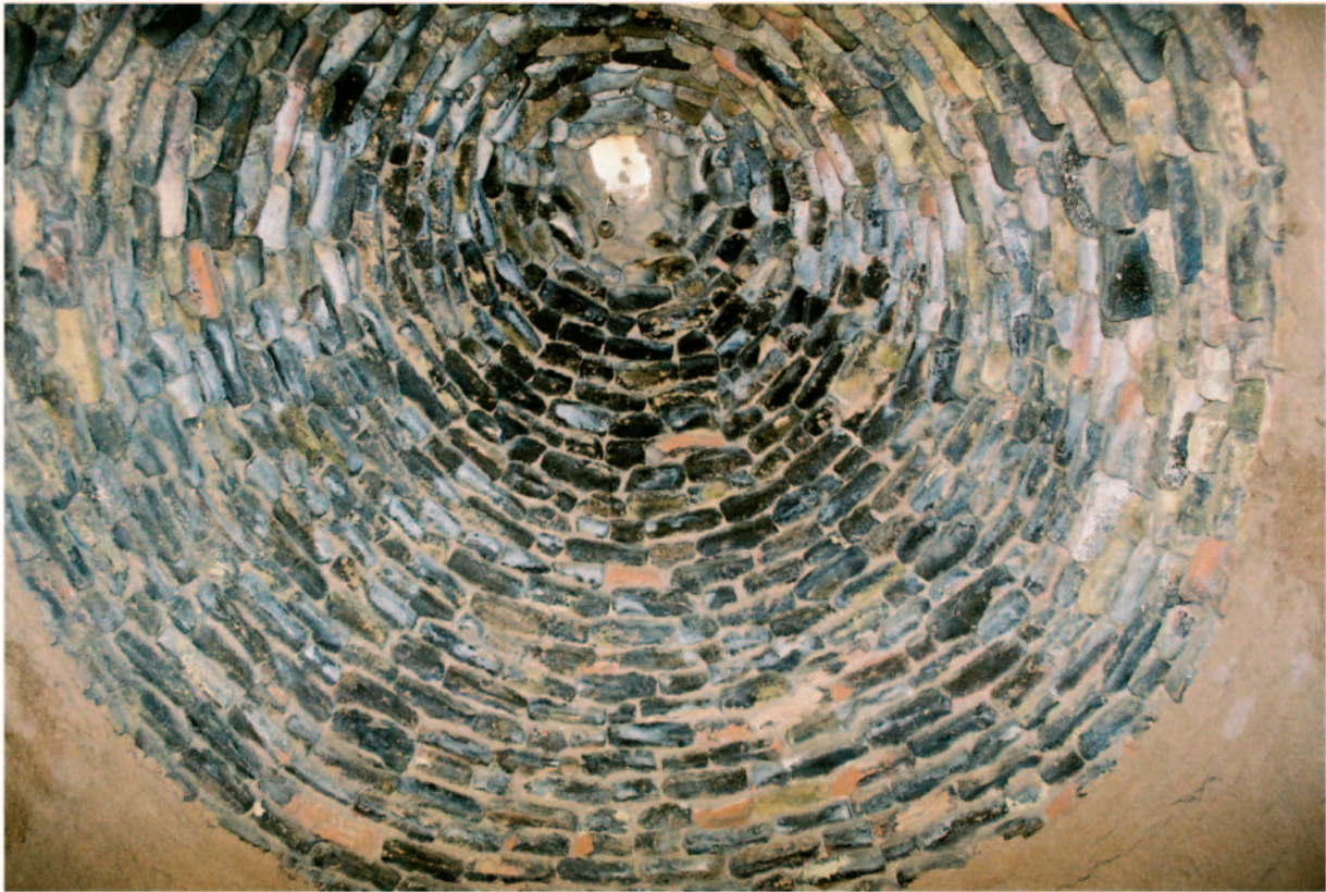
Fig. 2. Internal view of the dome in a Harran house.
