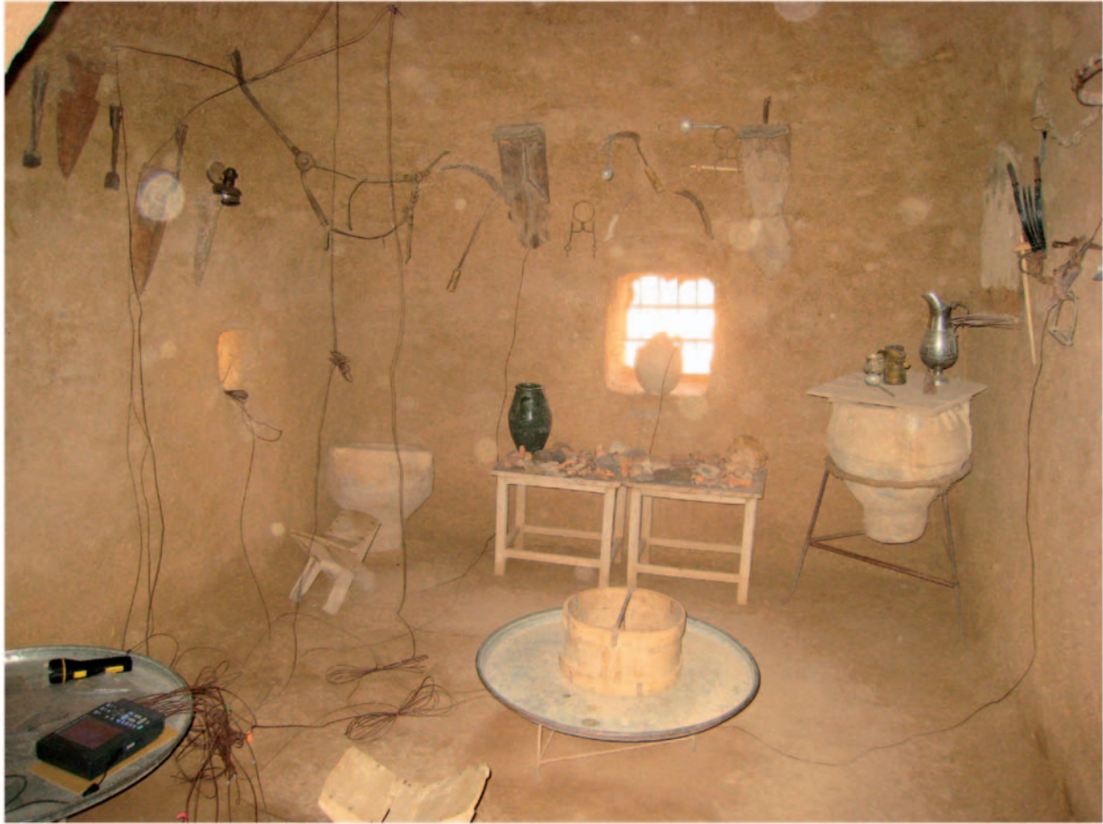
Fig. 6. Inside view of the domed house numbered 8 showing some of the placed thermocouples and HIOKI 8421-51 memory hilogger unit.
