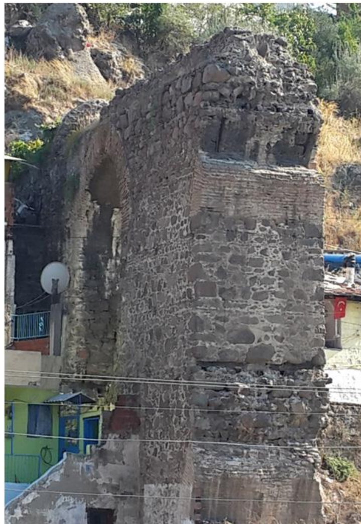
Figure 15. East elevation and demolished arches of wall portion B.
