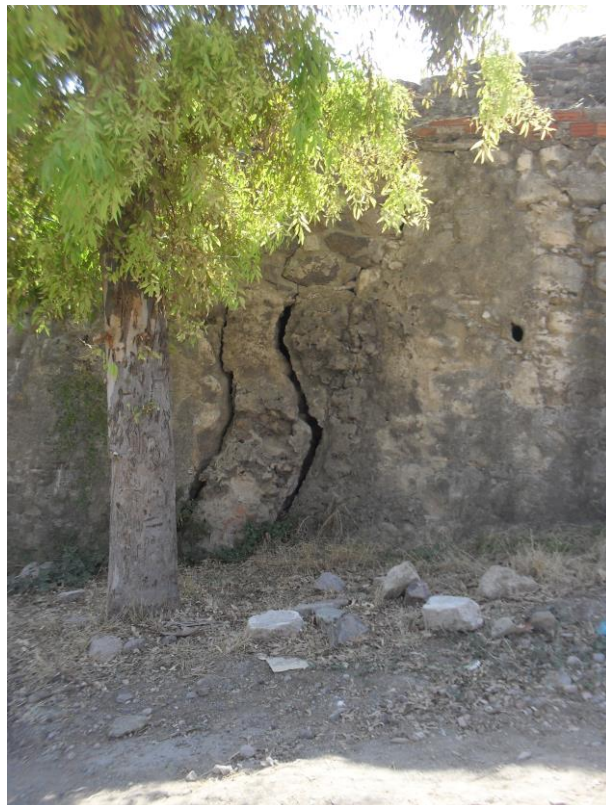
Figure 25. The fracture on wall portion A.
