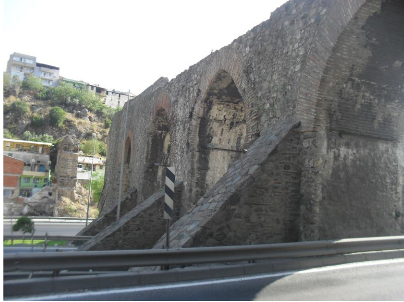
Figure 18. Three buttresses on east elevation.
