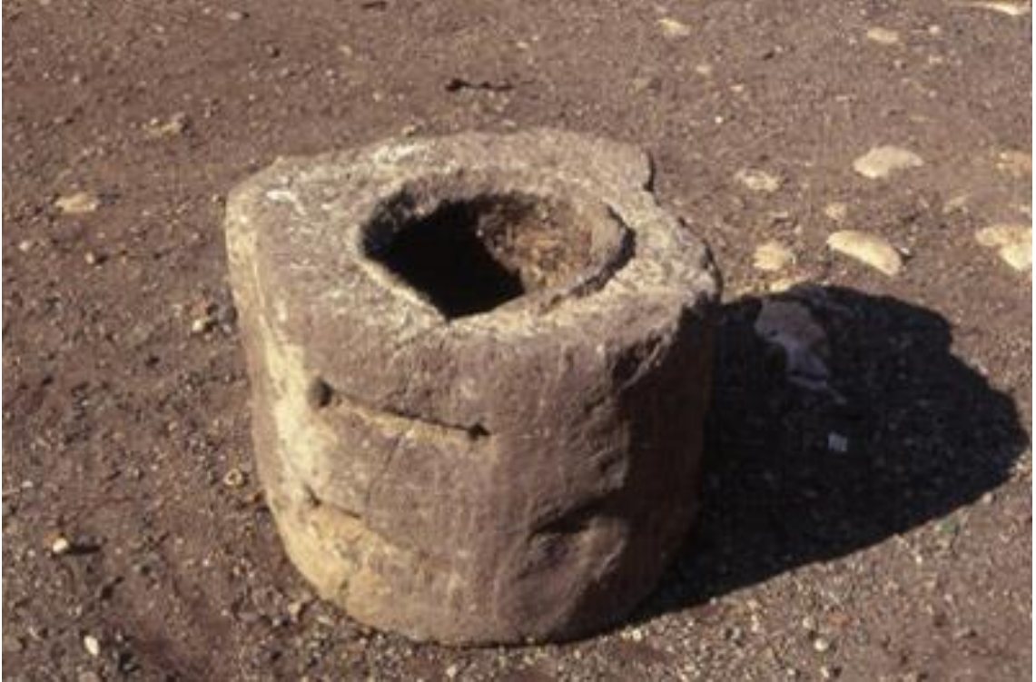
Figure 65. The remains of pipes of Karapınar Waterline. (Source: Öziş, et al., 1999)
