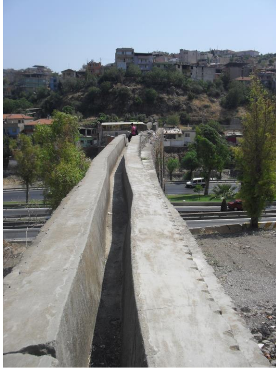
Figure 22. Concrete covered stone duct above wall portion A.
