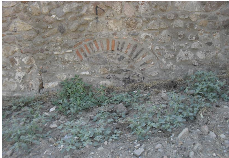
Figure 17. One of two blind arches on east elevation of wall portion A.
