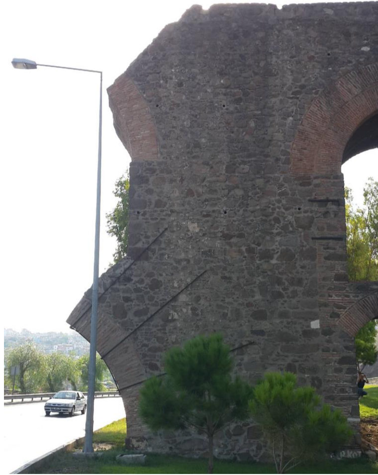
Figure 19. Three of six iron bars used to support remaining arches.
