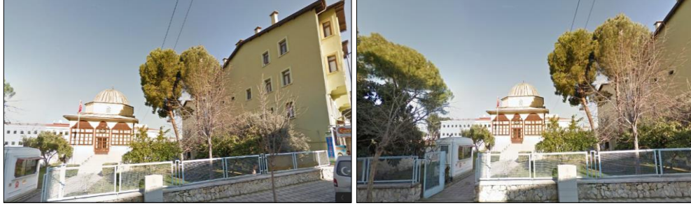
Figure 4.2. Surroundings of the Library (Source: GoogleMaps, 2016)
