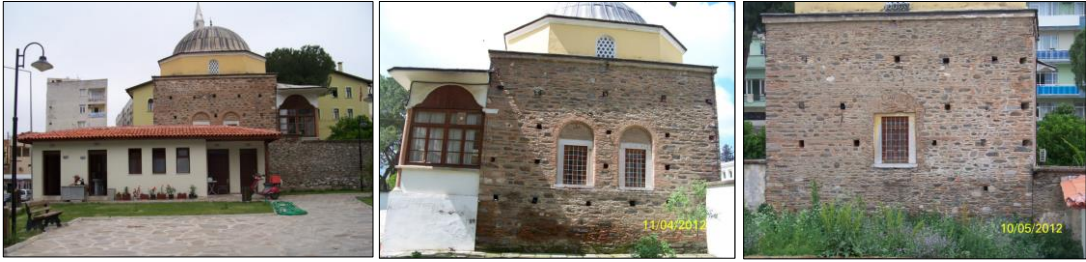
(a) (b) (c) Figure 4.3. Façades of the Library; (a) west (b) east and (c) north (Source: Ekizoğlu, 2012)
