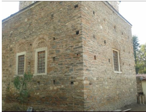
Figure 4.11. External walls of the Library
