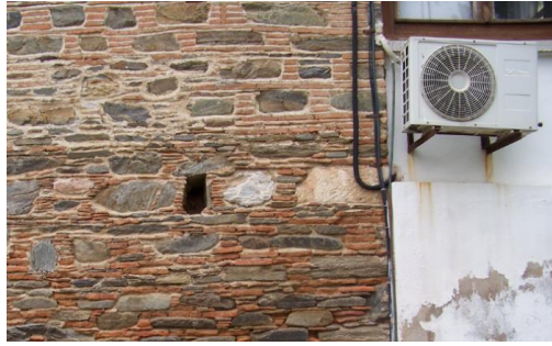
Figure 4.17. Split air conditioner used in the entrance zone of the Library (Source: Ekizoğlu, 2012)
