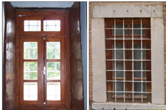
Figure 4.14. The configuration of windows (Source: Ekizoğlu, 2012)
