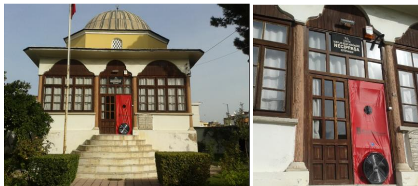
Figure 4.16. Blower door test and the configuration of sheeting covered door to the entrance door
