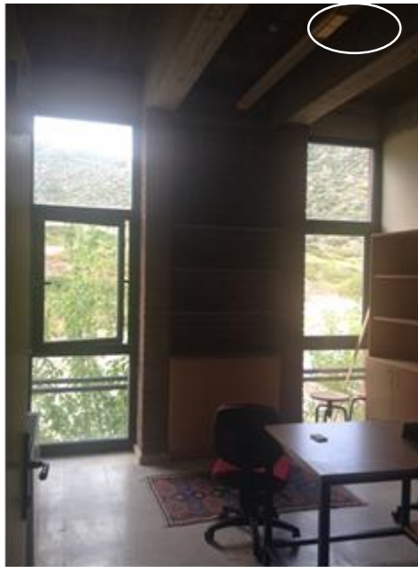
Figure 3.20. Location of the occupancy/light sensor.
