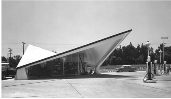
Figure 1 Hypar concrete shell.
