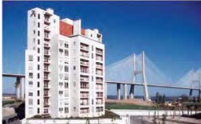
Figure 4.1. Concrete Building in Portugal [57].
