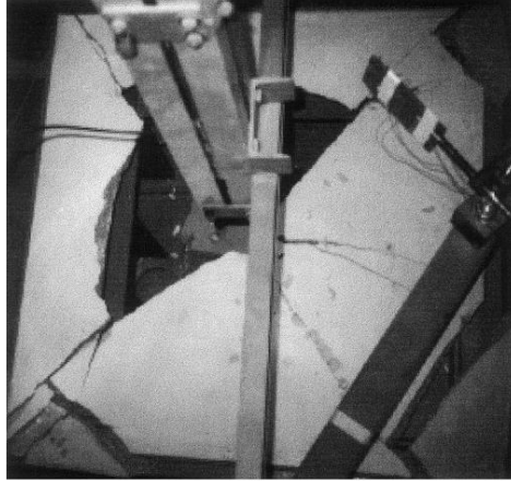
Figure 2.5. Failure of plain concrete slab (Source: Ong et al., 1999)
