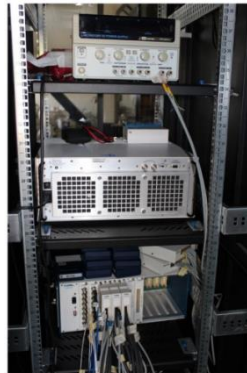
Figure 3.17. General view of Data Acquisition System
