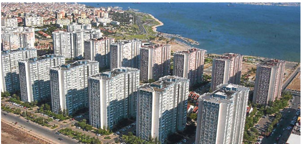
Figure 5.10. View of Mavişehir I Pamukkale high rises from air. (Source: Milliyet 2013)
