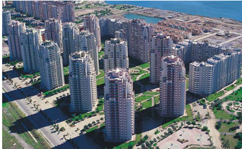
Figure 5.12. View of Mavişehir II Flamingo. (Source: Peyzajuygulama 2013)
