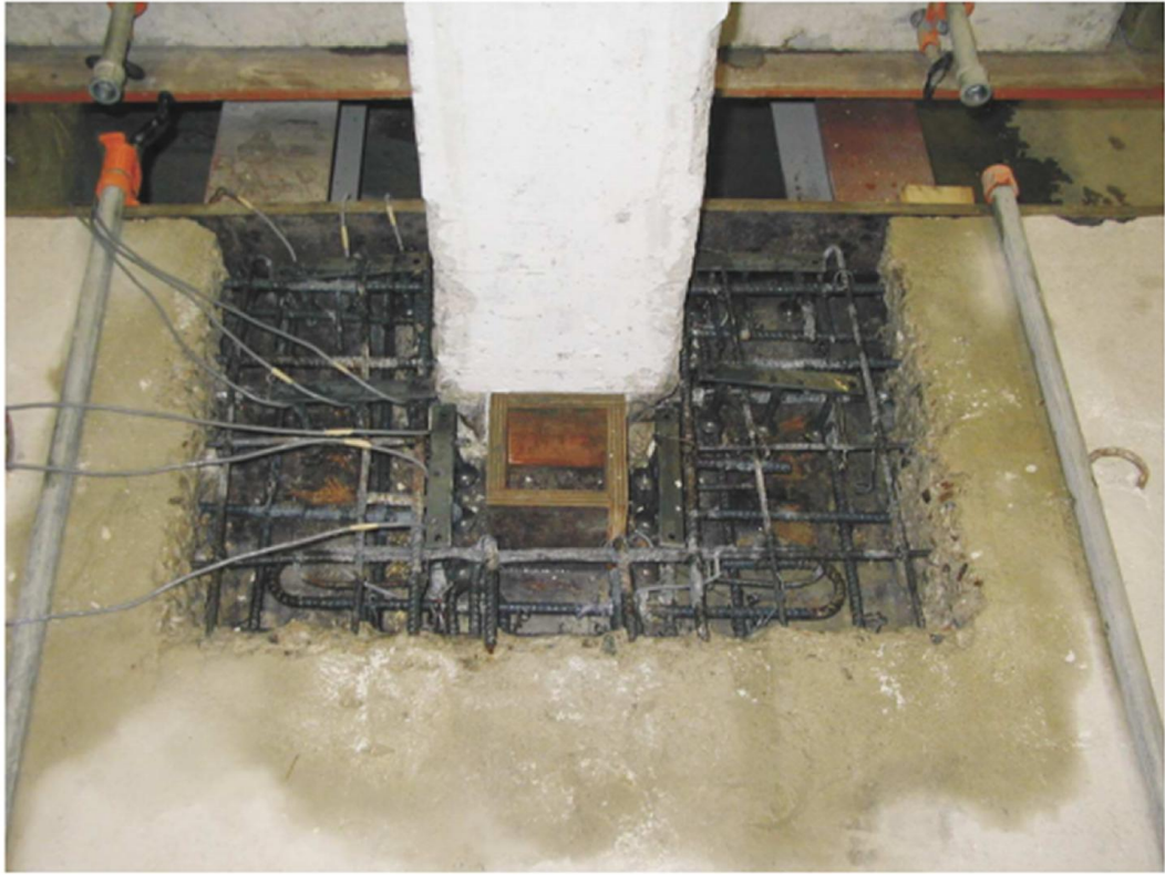
Figure 2.14. Removing the damaged concrete (Source: El-Salakawy et al., 2002)
