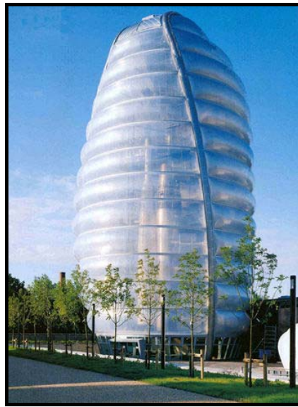
Fig.4. 22. External View Of NSSC (1) Source: www.skyspan.com
