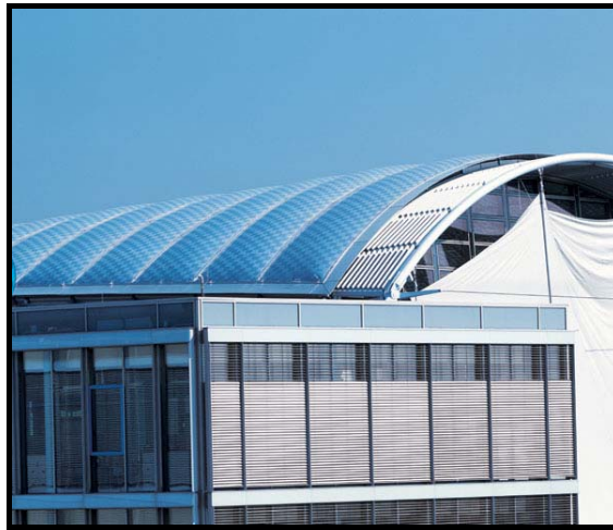
Fig.4. 17. External View Of Festo Technology Centre Source: www.pfeifer.de
