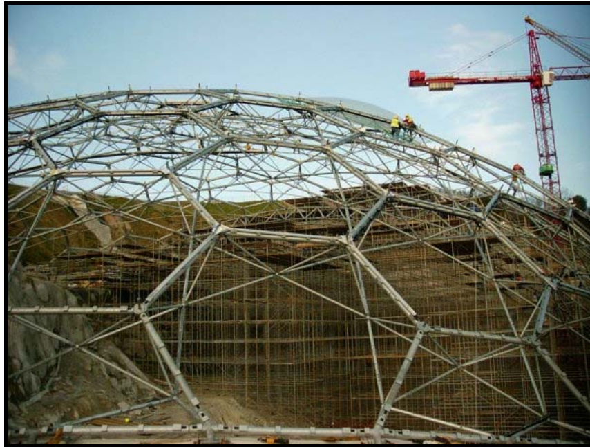
Fig.4.7. Construction Phase Of Eden Project (1) Source: www.edenproject.com
