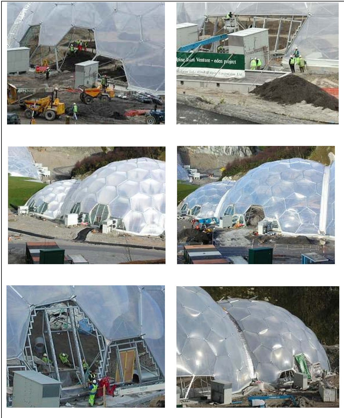
Fig. 4.2. Fan coils inflation equipments and ventilation blinds Source: www.eden-project.co.uk
