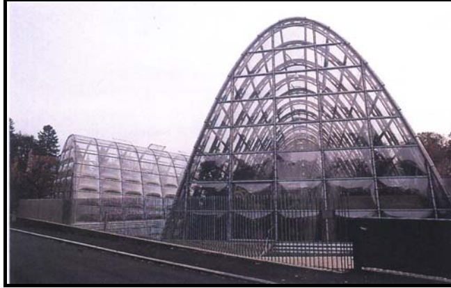
Fig. 3.5. Graz Greenhouse by Volker Giencke Source: Architectural Review, 1996/10
