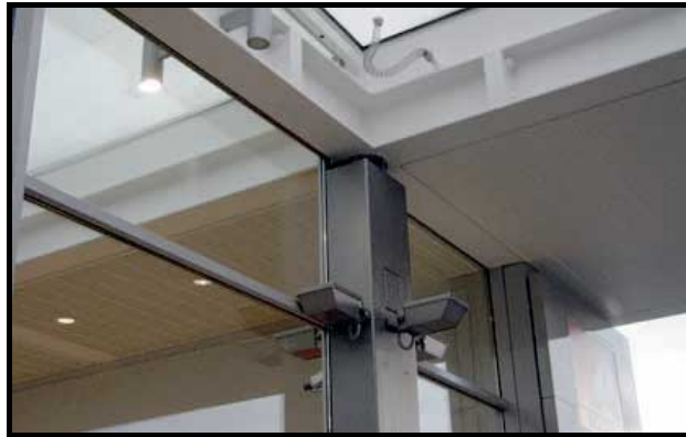
Fig. 3.28. Allgut Petrol Station Close Up Source: Haack and Höpfner Architects, 2003
