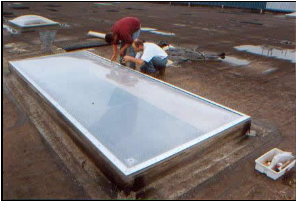
Fig. 3.52. Application Of IPS As A Skylight Source: www.buitink-technology .com
