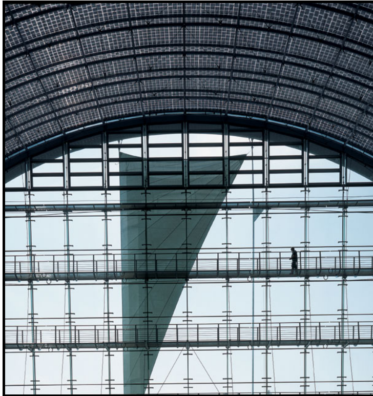
Fig. 4.18. Festo HQ Roof Close Up (1) Source: www.vsp.com
