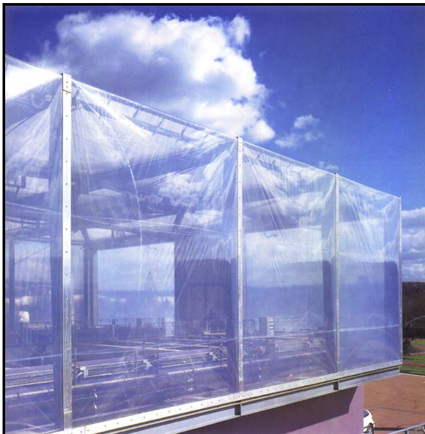
Fig. 3.33. Earth Center External View IPS Close Up Source: Detail, 2000 / 6
