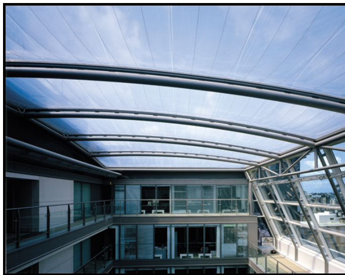
Fig.5.6. Adastral Houses High-Tech Atrium lets the noise out, Warner Bros. Source: www
