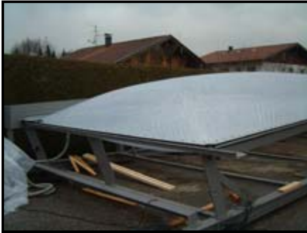
Fig. 3.25. Installation and Clamping Of Pillow System Source: www.buitink-technology.com
