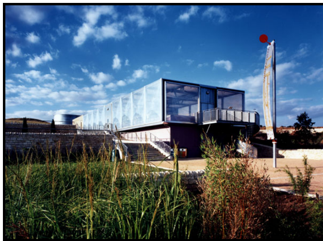
Fig. 3.39. Waterworks Pavilion at Earth Center, Doncaster Source: Detail, 2000/6
