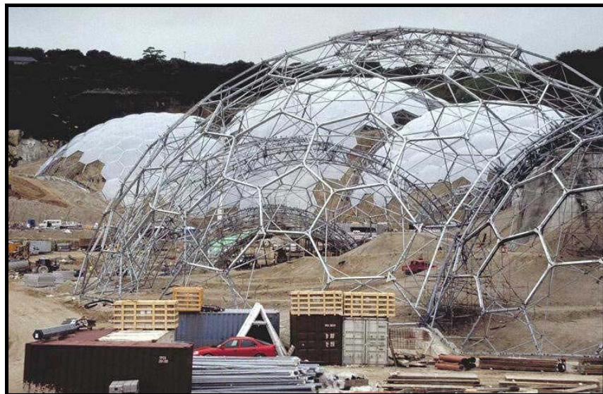
Fig.4.8. Construction Phase Of Eden Project (2) Source: www.edenproject.com
