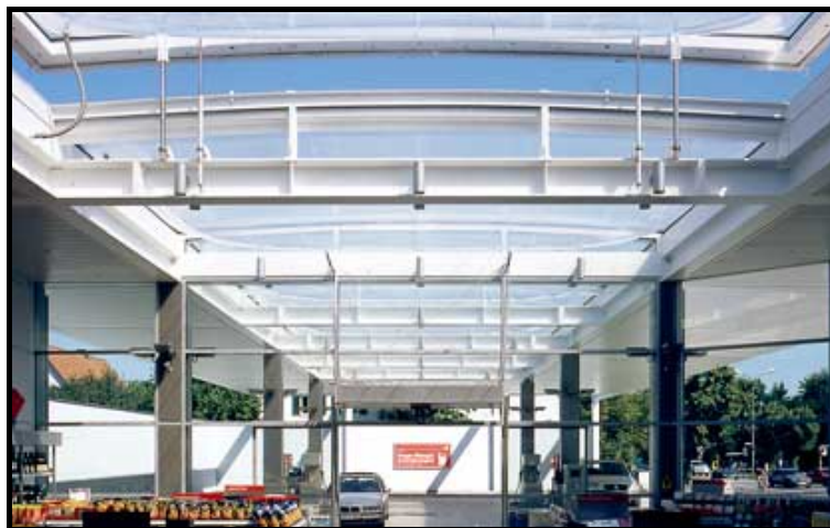
Fig.5.4. Allgut Petrol Station Canopy Source: Haack + Höpfner Architectural Firm website
