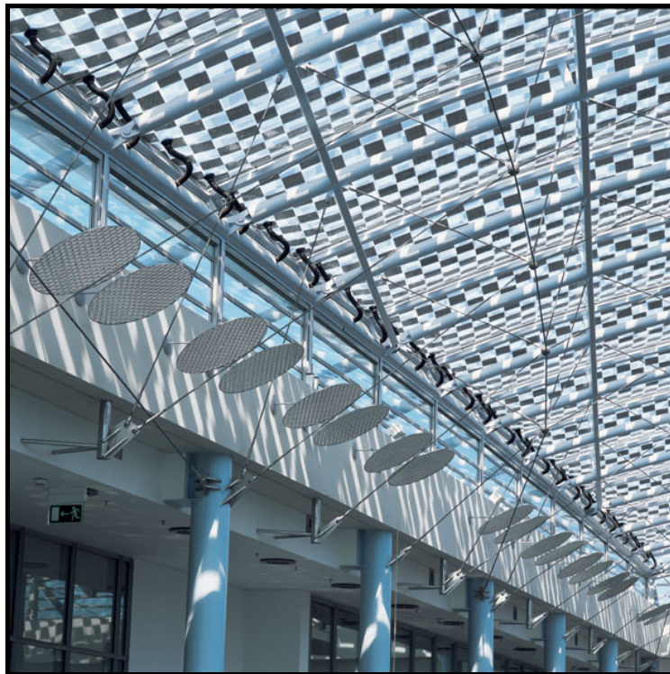
Fig. 4.19. Festo HQ Roof Close Up (2) Source: www.vsp.com
