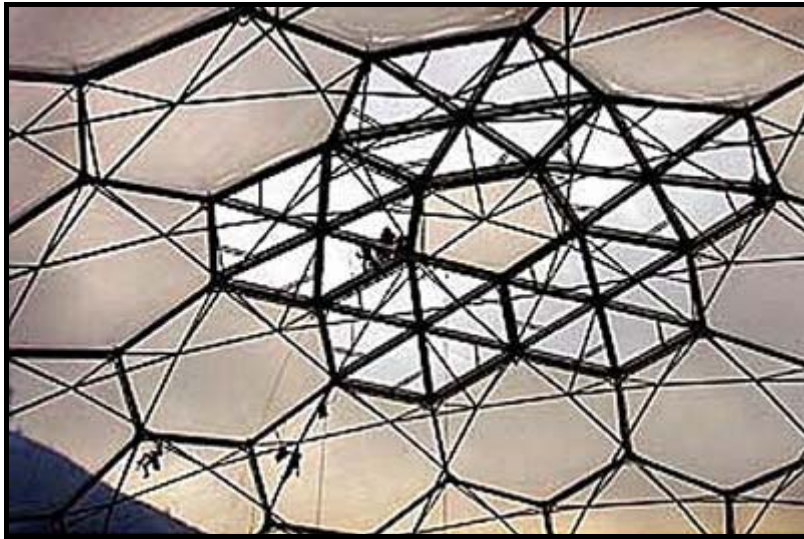
Fig.3.21. Workers Installing Etfe Foil Panels In The Dome Ceiling Source: www.apexphoto.com
