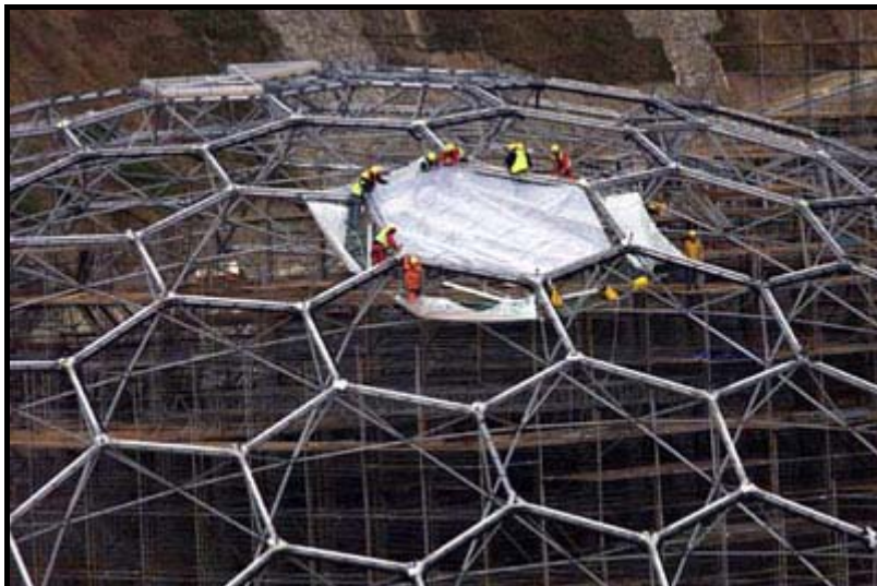
Fig.3.22. Each ETFE pillow is secured in the steel framework Source: www.apexphoto.com
