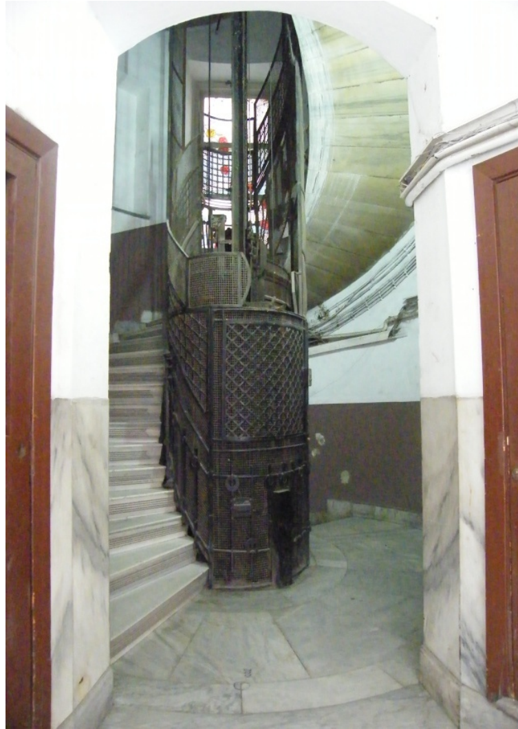
Figure 6. Original elevator of Botter Apartment
