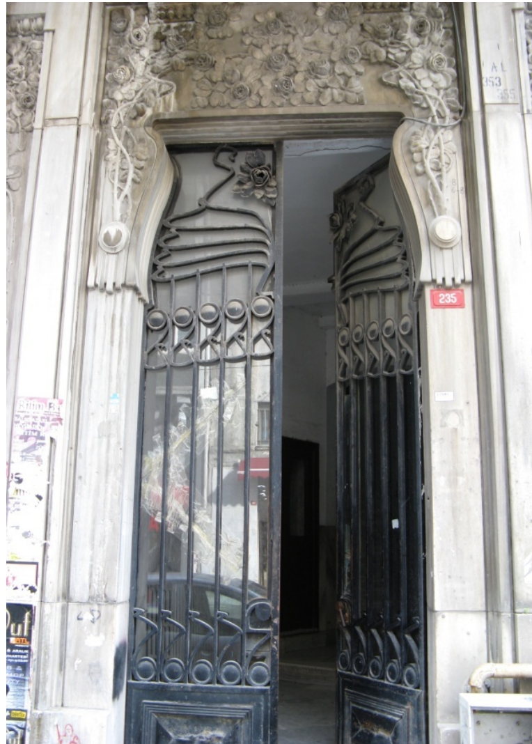
Figure 5. Florally ornamented main entrance door of Botter Apartment
