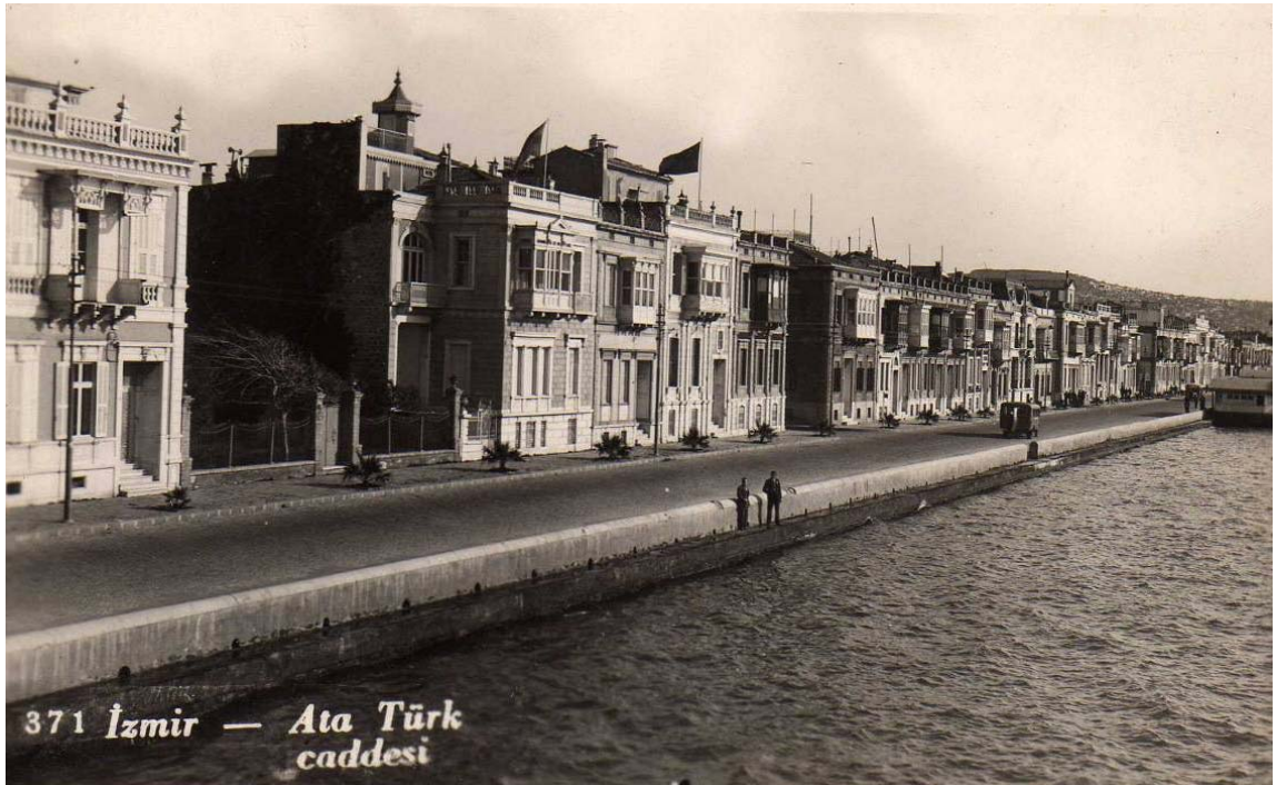
Figure 2.11. Consulate Building – 1920-1930's (Source: Arch.Cengiz Onaran's Archives)
