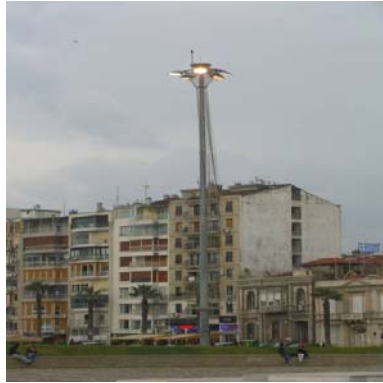
Figure 3.23 Example of Lighting Equipment
