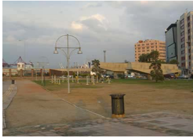
Figure 3.164. Neglected Landscaping in the Fitness Area
