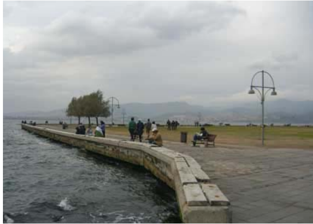
Figure 3.52. Side Seating on Parapet
