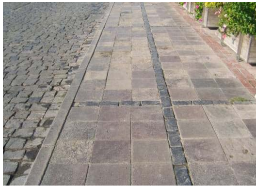
Figure 3.7. Pavement on Sidewalk
