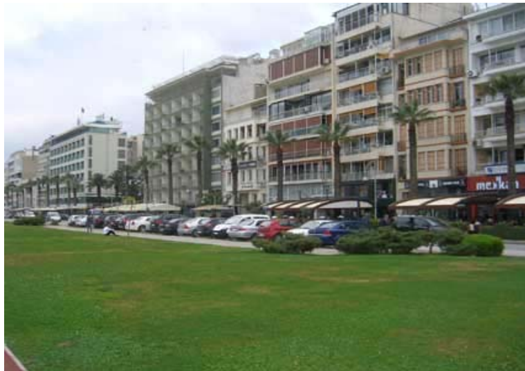
Figure 3.73. Landscaping and Car Parking
