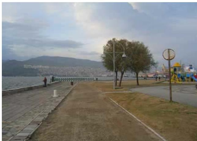
Figure 3.162. Neglected Walking Path and Landscaping
