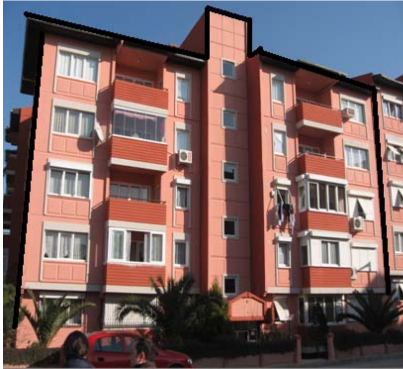
Figure 5.6. Southwest (entrance) façade of the apartment block
