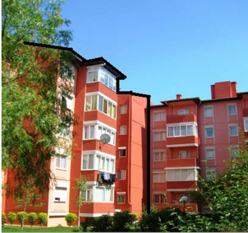
Figure 5.8. Northeast façade of the apartment block facing the courtyard
